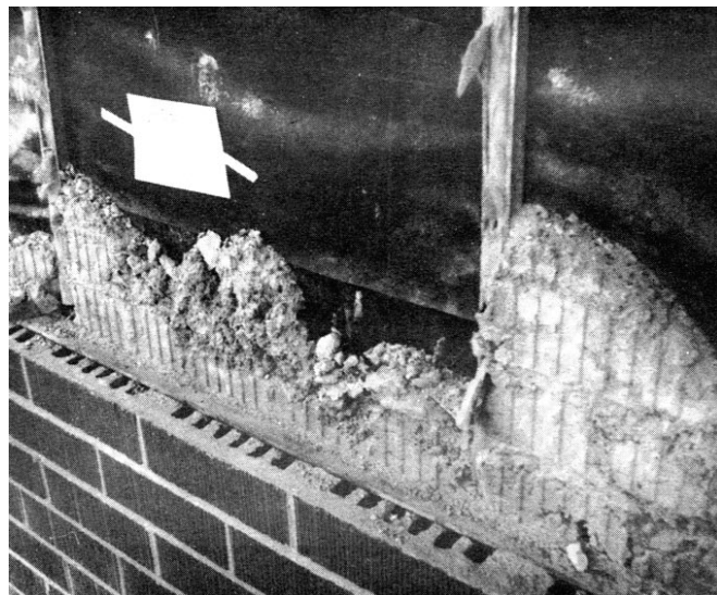
Figure 3. The cavity behind the brick veneer is clogged with mortar, trapping moisture and holding it against the stud wall.
