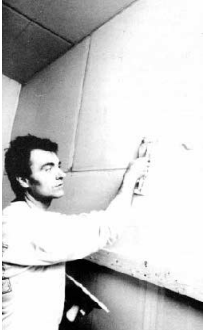
Drywall finisher Smokey Lyons trowels on the finish coat of mud over Gypsonite . Because of plasticizers in the mud, it has a dough-like consistency, which takes some getting used to. The edges of Gypsonite boards are beveled on all four sides (right). This simplifies joint finishing, but also makes the corners fragile.
