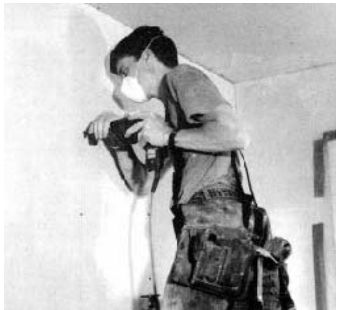
A 3 1/2-inch Makita cordless saw with carbide blade (above, left) worked well for cutting narrow pieces, but strained the saw and ran down the battery. Hanging the board was routine (above), but required a bit more force behind the screwgun and a full-depth adjustment to set the heads. The sheets are installed with a gap to ensure a good edge bond for the adhesive that glues the sheets together (left).
