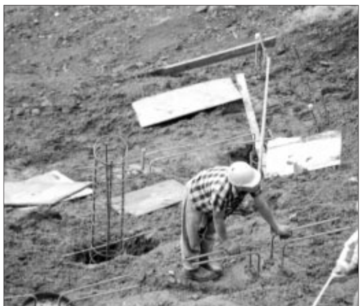
Figure 4. Use half sheets of plywood to protect pier holes from contamination by loose dirt and to prevent workers from falling in. Pour concrete to grade in the pier holes; the exposed rebar connections will be poured later as part of the grade beams and retaining walls.
