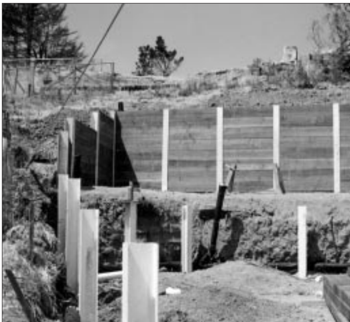
Figure 2. This I-beam shoring design uses pressure-treated timbers between soldier piles anchored in concrete. Some require steel tie-backs that work like toggle bolts screwed into the hillside to hold the wall in place.
