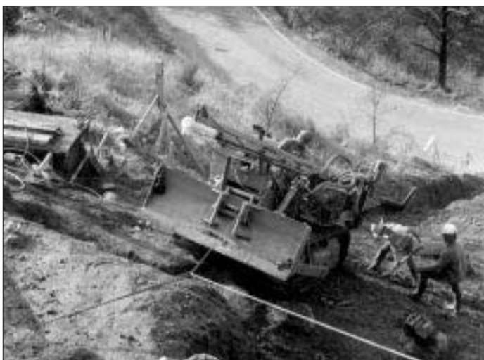
Figure 3. Site access is crucial in determining the type of machine you use to drill piers. Most pier drillers attach to a steel cable and lower themselves onto the site with a winch.
