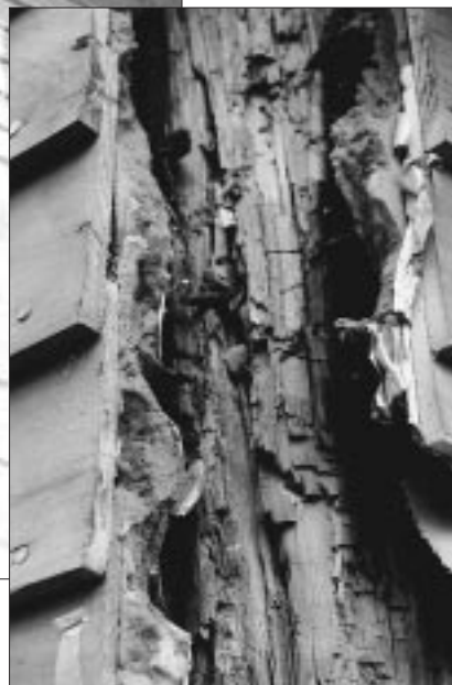
Brown rot blues. After only four years, the corner post of this house shows extensive damage from brown rot (right). The cause: excessive moisture trapped behind foil-faced foam board applied to the exterior.
