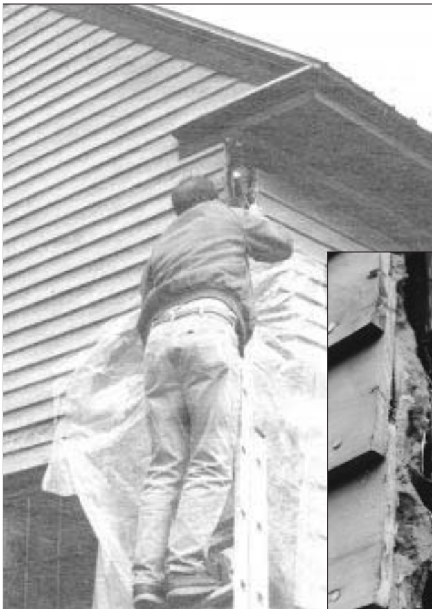
Brown rot blues. After only four years, the corner post of this house shows extensive damage from brown rot (right). The cause: excessive moisture trapped behind foil-faced foam board applied to the exterior.
