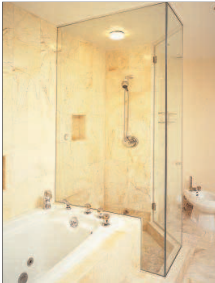
Figure 3. For a unique look, glass shower panels can be custom-cut at the factory, but such installations require precise field measurements.
