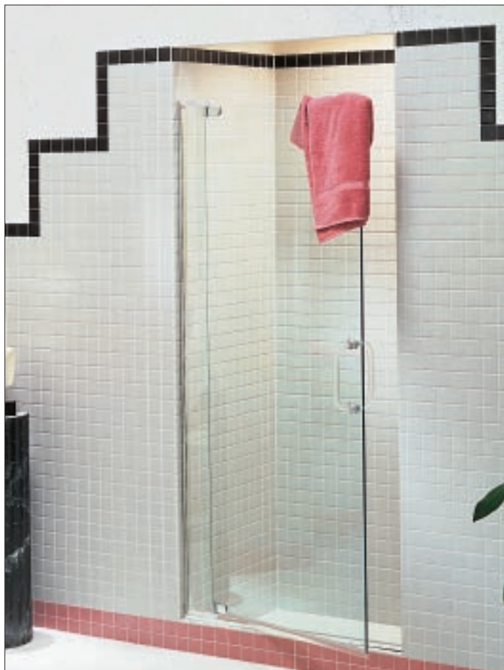
Figure 4. When remodeling a shower, the author often removes the low ceiling and narrow jambs, and installs clear glass to create a modern, open look.
