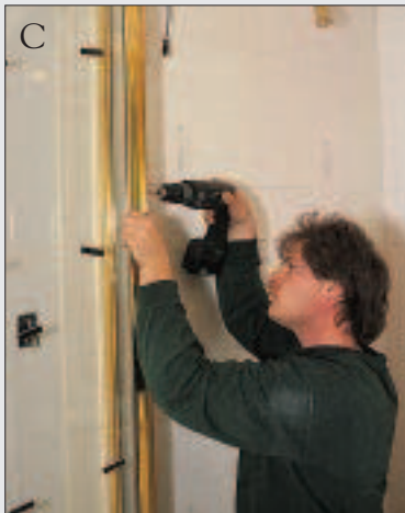
High-quality extrusions, like these by Century Shower Door, fit snugly together, allowing the installer to friction-assemble the unit (A) and adjust the reveals where necessary (B). After carefully drilling holes in the metal components (C), the author screws the unit together (D).
