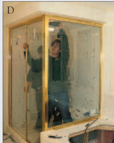
High-quality extrusions, like these by Century Shower Door, fit snugly together, allowing the installer to friction-assemble the unit (A) and adjust the reveals where necessary (B). After carefully drilling holes in the metal components (C), the author screws the unit together (D).
