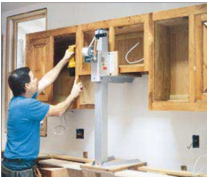
Figure 2. Using the alternate base, the author installs upper cabinets after the base cabinets are in place.
