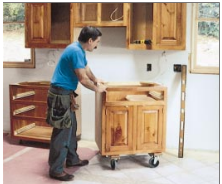
Figure 3. The base of the Gil-Lift can be used as a dolly to maneuver base cabinets into place.
