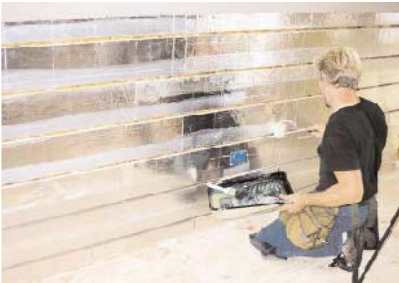
A paint roller is used to apply contact adhesive to foil-faced foam before mounting aluminum heat-transfer plates. Adhesive is used only on one edge of each strip to allow for thermal movement.
