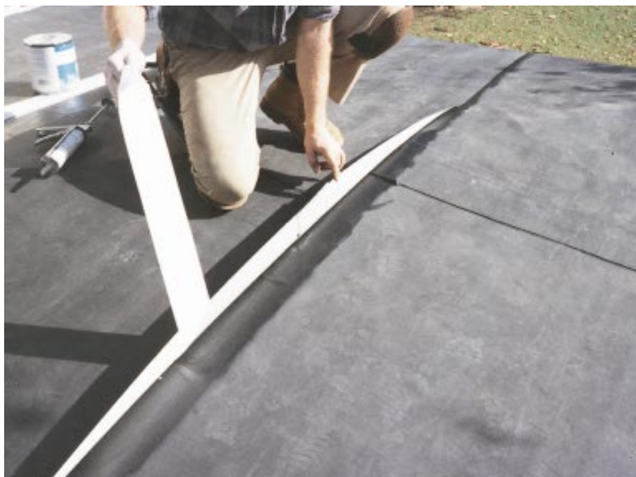
Figure 5. With all of the courses installed, the author goes back and prepares the overlaps with primer before peeling off the 4-inch-wide protective strip and bonding the edge. A vigorous follow-up treatment with a wood or steel seam roller assures a good seal without bubbles or blisters.
