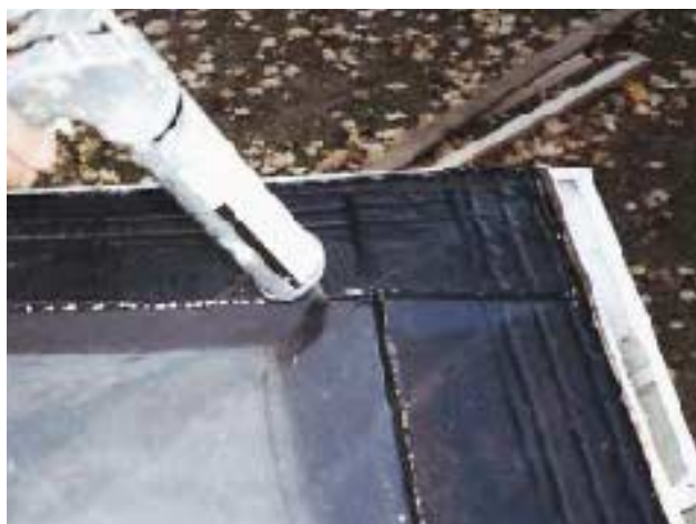
Figure 9. Perimeter drip edge and all membrane seams are covered with a cover strip, made of the same pliable material as the corner seal (above). Sealant, applied to all exposed edges of the cover strip, completes the job (right).
