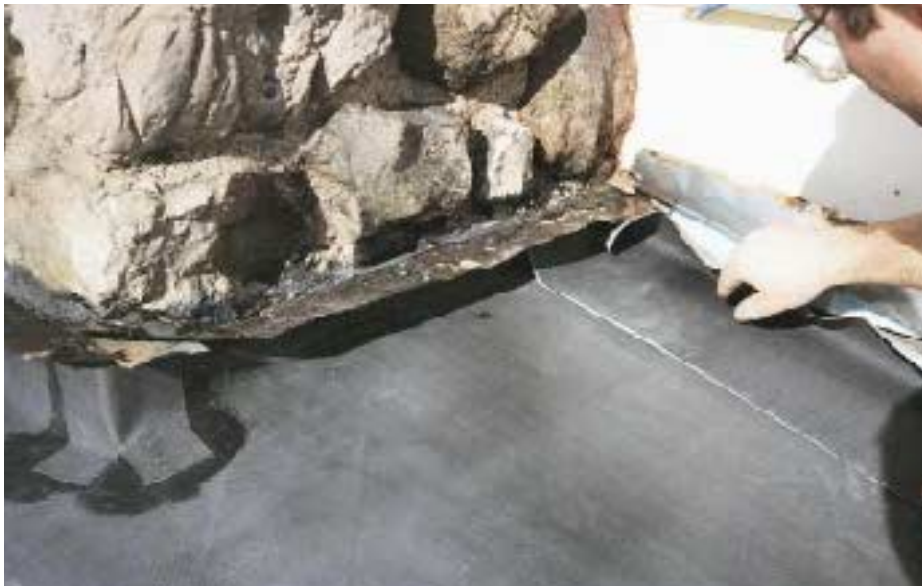
Figure 6. The membrane should self-flash as high up an abutting wall as possible. In this case, existing metal flashing at the chimney and sidewall restricted the vertical return. The author used a putty knife to coax the membrane into place under the metal (top). The membrane folds into inside corners; outside corners are slit to make the transition, then reinforced with a small patch of roofing material bonded over a primed surface (above).
