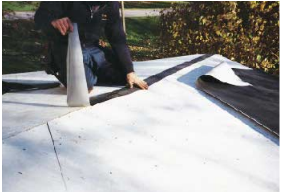
Figure 1. Weatherbond 110 self-adhering EPDM must be installed over a clean, paint-primed substrate. The author paints OSB sheathing prior to installation in order to speed the membrane installation. To protect the membrane from wear over sharp corners, he installs a 6-inch-wide strip of the membrane over the transitions first.
