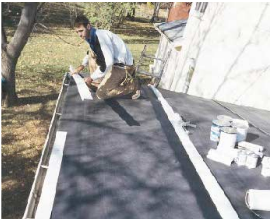
Figure 3. A standard 2½-inch-wide aluminum drip edge is installed over the membrane to provide a clean-looking perimeter and direct water into the gutter. An EPDM cover strip will be applied later to seal the material transition.
