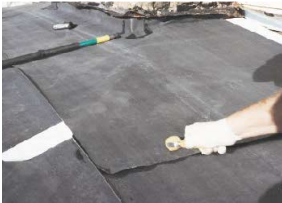
Figure 4. Splices in a course must be prepared with a proprietary primer before joining with a minimum 4-inch overlap. Peeling back a short length of the separate 4-inch-wide parting strip along the bottom edge allows full-width bonding of the splice.
