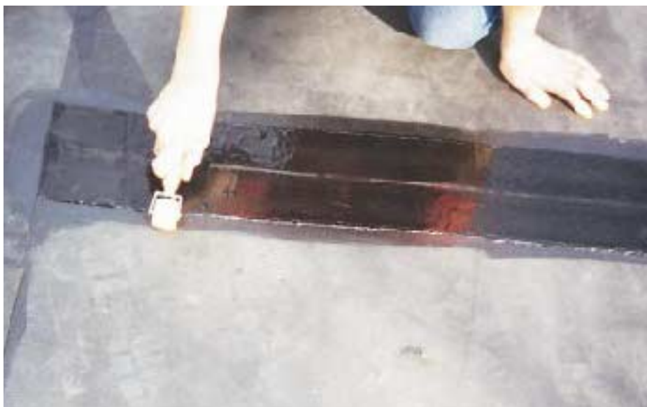
Figure 9. Perimeter drip edge and all membrane seams are covered with a cover strip, made of the same pliable material as the corner seal (above). Sealant, applied to all exposed edges of the cover strip, completes the job (right).
