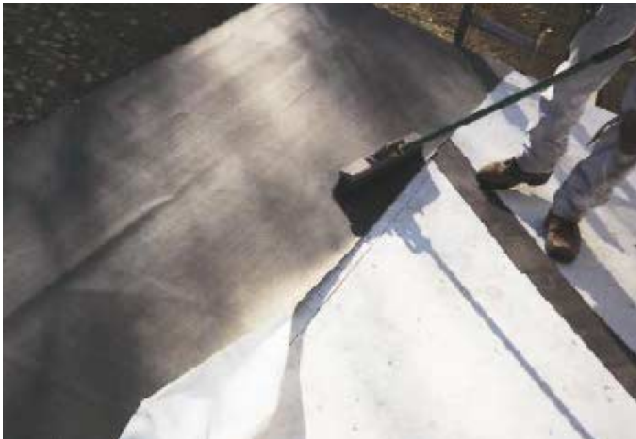
Figure 2. The starter course overhangs the roof edge by about 1½ inches. A push broom is the ideal tool to embed and smooth the membrane into place as the protective paper facing is peeled away.
