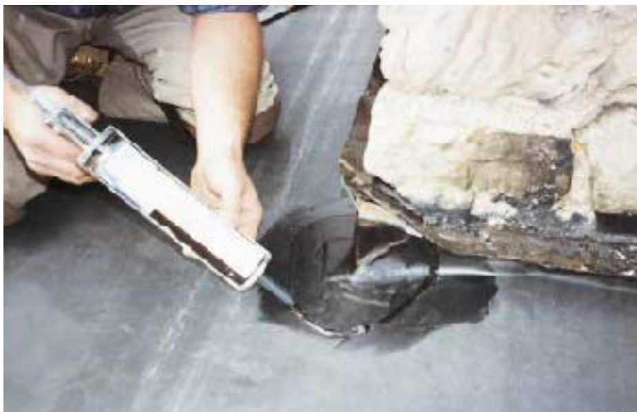
Figure 7. A proprietary corner cover, made of a more pliable EPDM rubber, can be readily stretched and formed to protect inside and outside corner transitions from roof to wall (top). As with all rubber-to-rubber bonds, it's necessary to prime the surface of the bonding area first. All cover edges receive a continuous bead of system sealant, feathered while wet to knock down the ridges (above).
