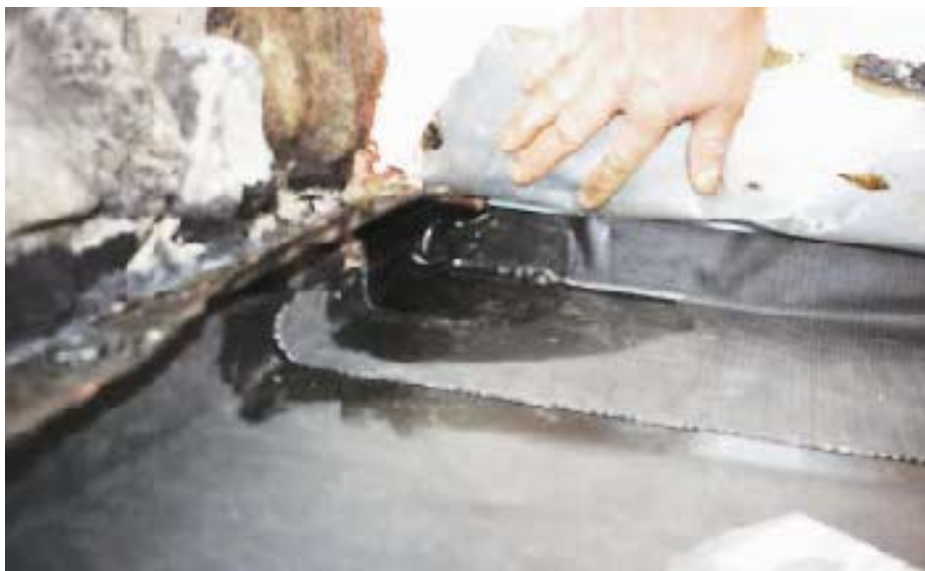
Figure 8. An outside corner is fairly simple to install; trickier inside corners follow a prescribed sequence of folds to install properly. Leftover material is folded onto itself and all edges are caulked with proprietary sealant.
