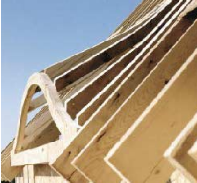
The window frame is a sandwich of 2-by stock and \frac{3}{4} -inch plywood, both cut with a router and template. The curved rafters were cut from clean 2x12s.
