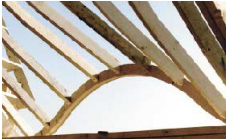
The window frame is a sandwich of 2-by stock and \frac{3}{4} -inch plywood, both cut with a router and template. The curved rafters were cut from clean 2x12s.
