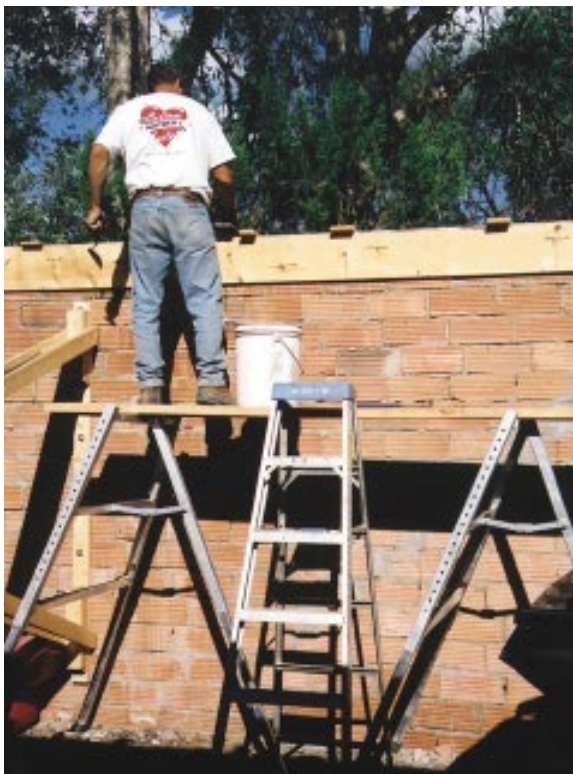
Figure 1. At its maximum height, which is still less than 72 inches, no fall protection is required with Bronco scaffolding.
