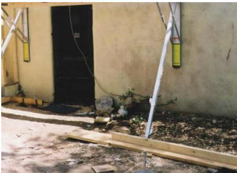
Figure 4. The MonoJack is easy to set up and provides a working platform up to 16 feet high, with a minimal footprint on the ground.
