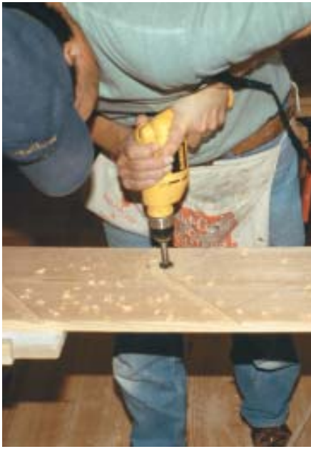
Figure 6. A Forstner drill bit outlines the nosing profile on the housed stringer. The housings are completed with a wobble-dado blade in a radial-arm saw and cleaned up with a straight bit in a hand-held router.
