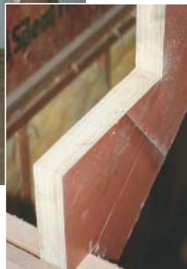
Figure 1. Although rough stringers are seldom perfect, LVL stringers (inset) are far less prone to shrinkage distortion and are useful for spanning exceptionally long stair flights.
