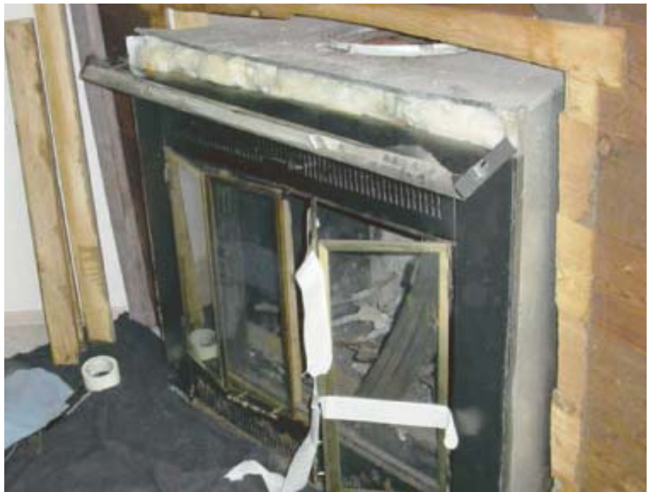
Figure 4. The simple three-board facing around this circulating fireplace was easily removed without damage, making it possible to slide it forward into the living space for removal.
