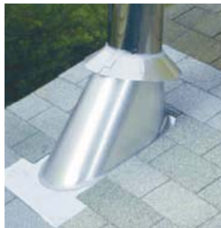
Figure 9. In applications where the flue exits through the roof, the penetration can be enclosed in a site-built or manufactured rooftop chase or left exposed and weatherproofed with a standard flashing kit, shown here.
