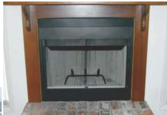
Figure 6. Gaps between a smaller replacement fireplace and the existing interior finish (left) are closed with a custom sheet-metal surround screwed to the front of the fireplace (below). Existing assembly screws on the fireplace are backed out enough to allow the notched flange of the surround to slip into place before being tightened down with a nut driver (below left). Where needed, extended trim is added to the sides of the fireplace as well.
