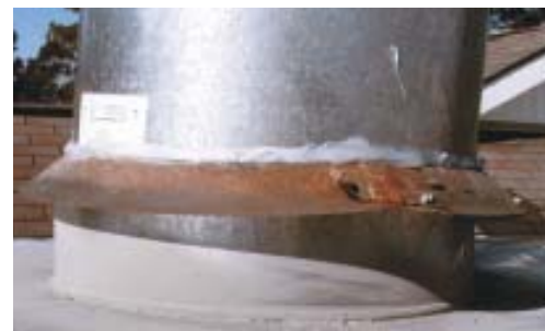
Figure 8. The stamped one-piece chase covers provided by many fireplace manufacturers are a common source of leaks (left). The author's preferred cover, fabricated by a local sheet-metal shop, has a soldered collar that extends several inches above the cover itself (below). A conical storm collar is caulked to the flue with silicone. The cover is sized to extend an inch beyond the chase on all sides to prevent water that drips from the edges from running down the outside of the chase and rotting the siding.
