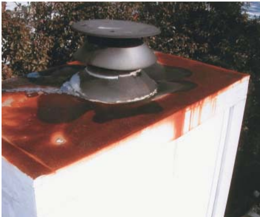
Figure 8. The stamped one-piece chase covers provided by many fireplace manufacturers are a common source of leaks (left). The author's preferred cover, fabricated by a local sheet-metal shop, has a soldered collar that extends several inches above the cover itself (below). A conical storm collar is caulked to the flue with silicone. The cover is sized to extend an inch beyond the chase on all sides to prevent water that drips from the edges from running down the outside of the chase and rotting the siding.
