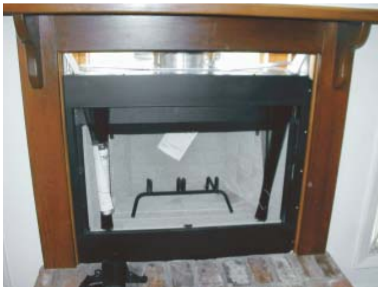
Figure 6. Gaps between a smaller replacement fireplace and the existing interior finish (left) are closed with a custom sheet-metal surround screwed to the front of the fireplace (below). Existing assembly screws on the fireplace are backed out enough to allow the notched flange of the surround to slip into place before being tightened down with a nut driver (below left). Where needed, extended trim is added to the sides of the fireplace as well.
