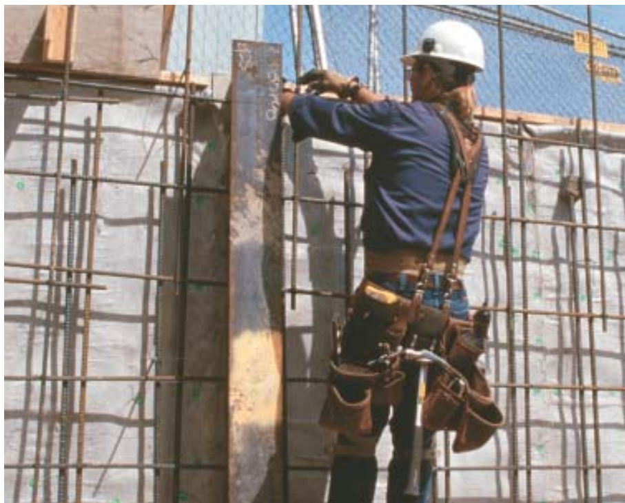
Figure 2. Highly tensioned guide wires are strung across the faces of the forms to control depth and permit accurate screeding. The steel soldier beam supports temporary shoring during construction (left). The vertical guide wire in this partially completed basement allows the finishers to create a sharply defined outside corner (right).
