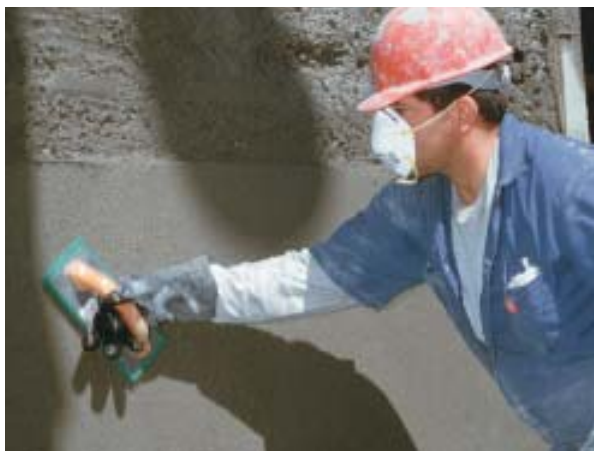
Figure 9. Shotcrete can be finished and ornamented in various ways, but a simple rubber-float finish is a common choice for utility applications.
