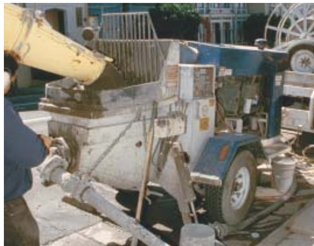
Figure 4. In addition to the ready-mix truck visible at rear (left), a shotcrete job requires a high-powered compressor mounted on a flatbed truck and a tow-behind concrete pump. The author's shotcrete sub brings a second concrete pump to the site as a backup. The batched concrete is discharged directly into the hopper of the pump and is then forced through a 2-inch hose to the nozzle, where compressed air is added (above).
