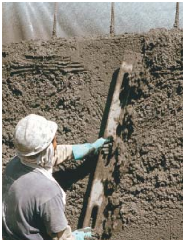
Figure 8. As each successive 3- to 4-foot lift of shotcrete is built to the required depth, it's screeded to the guide wires. The lift below has already been screeded and troweled; when the current lift has been finished the same way, the nozzleman will spray another lift over the exposed rebar visible at the top of the photo.
