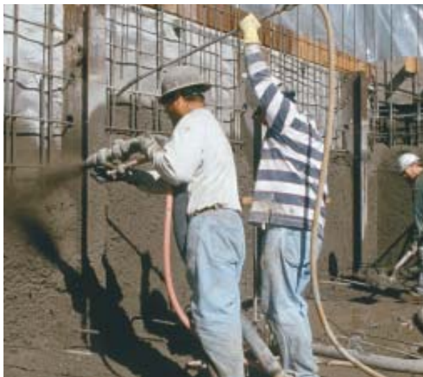
Figure 5. The shotcrete nozzleman guns a steady stream of concrete against a below-grade foundation wall while the blowpipe operator prepares to blow away unconsolidated debris, known as rebound. The area to the right has already been screeded to the level of the guide wires.
