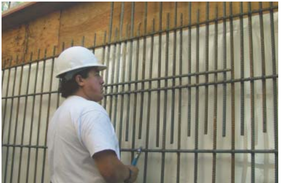
Figure 1. In this basement application, the lower part of the wall will be shot against the bank, which has been covered with a waterproofing membrane. The above-grade section is backed by a single-sided plywood form. To prevent the completed rebar grid from vibrating when struck by the high-pressure stream of shotcrete, the top will be wired to the plywood form and the bottom to rebar projecting from the floor slab. Number 2 wire chairs, not shown, will be wedged between the grid and the bank or form to maintain the proper spacing.
