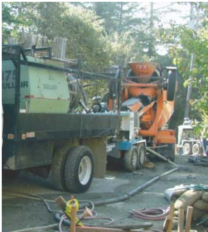
Figure 4. In addition to the ready-mix truck visible at rear (left), a shotcrete job requires a high-powered compressor mounted on a flatbed truck and a tow-behind concrete pump. The author's shotcrete sub brings a second concrete pump to the site as a backup. The batched concrete is discharged directly into the hopper of the pump and is then forced through a 2-inch hose to the nozzle, where compressed air is added (above).
