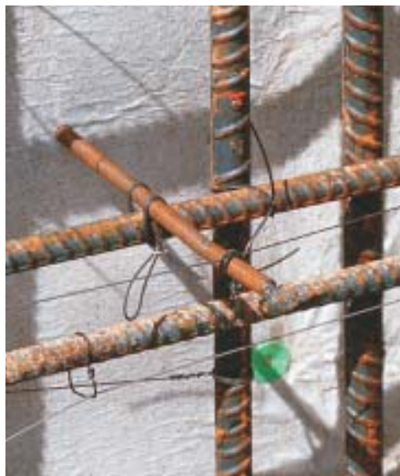
Figure 3. A length of threaded rod, driven through the bentonite-coated polyethylene waterproofing membrane and into the soil beyond, serves both to anchor the rebar grid and to position a horizontal guide wire that will help define the face of the finished shotcrete. The rod has been notched with bolt cutters so it can be snapped off after the wall has been sprayed and finished. To prevent leakage, the membrane penetration will be sealed with a proprietary mastic before the shotcrete is applied.
