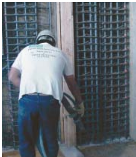
Figure 7. Heavily reinforced structural elements such as this pilaster are susceptible to shadowing and other defects if the shotcrete is applied improperly. To ensure quality, a mocked-up test panel is often shot, allowed to cure, and tested before construction begins.
