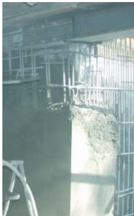
Figure 2. Highly tensioned guide wires are strung across the faces of the forms to control depth and permit accurate screeding. The steel soldier beam supports temporary shoring during construction (left). The vertical guide wire in this partially completed basement allows the finishers to create a sharply defined outside corner (right).
