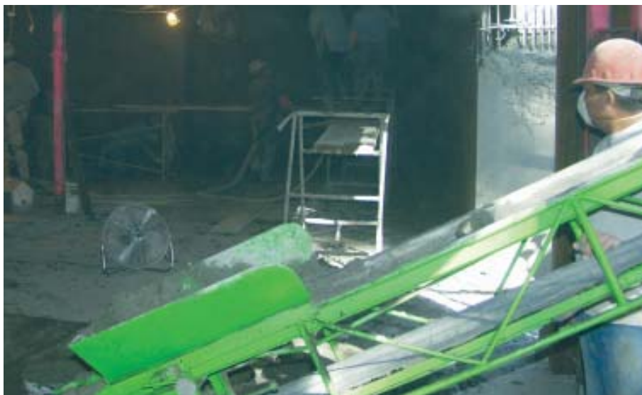
Figure 6. Up to 15% of the concrete used on a given job ends up as rebound, and several laborers may be kept busy removing this waste material. A material conveyor is an efficient way of moving rebound from a basement to ground level.
