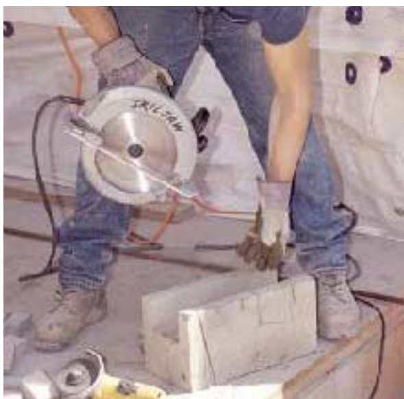
Figure 7. The walls between cells in standard 8-inch blocks are kerfed half-height with a masonry blade to create knock-out (KO) panels. A course of KO block allows rebar to be completely embedded in grout to form a bond beam.
