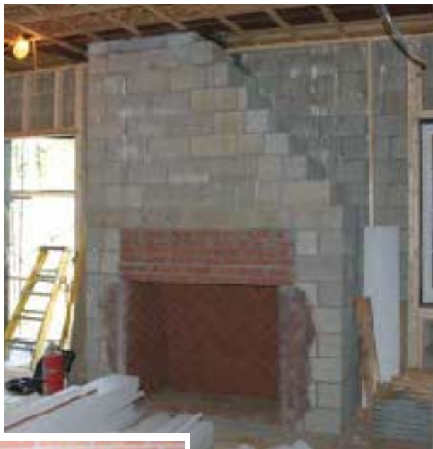
Figure 10. To end up in the center of the ridge three stories up, the flue has to staircase nearly 8 feet laterally (above). A series of structural pads, one at each floor, provides support for the stepped construction. A hand-laid herringbone brick pattern lends an artful touch to the fireboxes (left).
