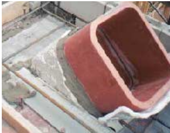
Figure 12. Shear anchors and rebar provide a mechanical connection among the steel, concrete, and masonry elements of the chimney. Cement board made a good leave-behind form for the slabs supporting the flue. Insulation wraps the flue tile to allow for thermal expansion.
