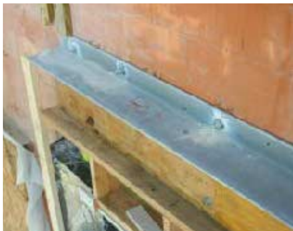
Figure 14. Galvanized steel lintels will support the exterior stone veneer above window openings. The lintel is bolted to the solidly grouted blockwork using epoxy-embedded anchor rods (right). Short lengths of steel lintel stairstep up the gables to support the finished stone veneer (below).
