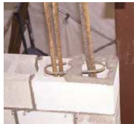
Figure 5. Stirrups bent from #3 rebar unify the effects of individual bars. Here, the stirrups circle two vertical rod pairs at a wall end, ensuring they will work in concert after the assembly is encased in concrete.
