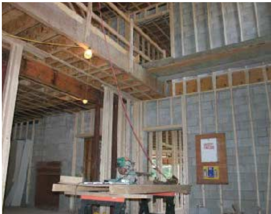
Figure 3. This massive block wall rises three stories from the basement level where it begins. LVL beams anchored into bond beams at each floor level support the joists, while the wall studs are nonbearing. One of the off-center fireplaces can be seen at lower left.
