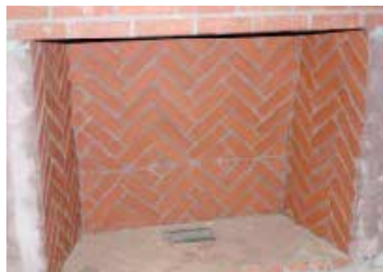
Figure 10. To end up in the center of the ridge three stories up, the flue has to staircase nearly 8 feet laterally (above). A series of structural pads, one at each floor, provides support for the stepped construction. A hand-laid herringbone brick pattern lends an artful touch to the fireboxes (left).
