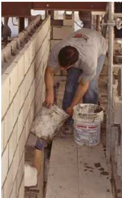
Figure 9. It took more than 30 yards of grout, passed up in buckets, to fill the block shear walls.
