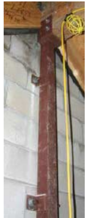
Figure 13. Epoxy-set Hilti HIT anchor rods secure LVL floor girders to the masonry. Asphalt felt provides a capillary break between wood and concrete (above). At right, a saddle-top steel post supports the ridge of a lower roof abutting the masonry gables.
