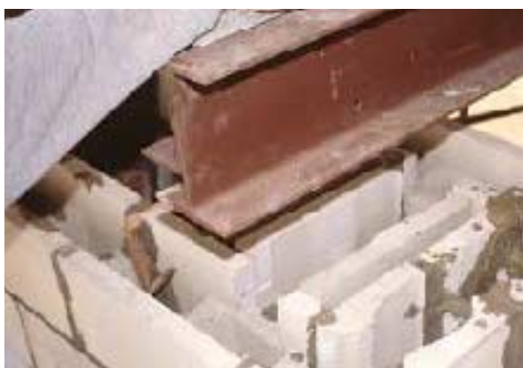
Figure 8. The chimney flue interrupts the bond beam running through the block wall at each floor level. To ensure the continuity of the load path, the bond beam encircles the flue.
