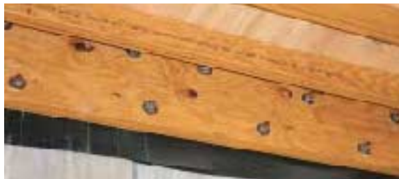
Figure 13. Epoxy-set Hilti HIT anchor rods secure LVL floor girders to the masonry. Asphalt felt provides a capillary break between wood and concrete (above). At right, a saddle-top steel post supports the ridge of a lower roof abutting the masonry gables.
