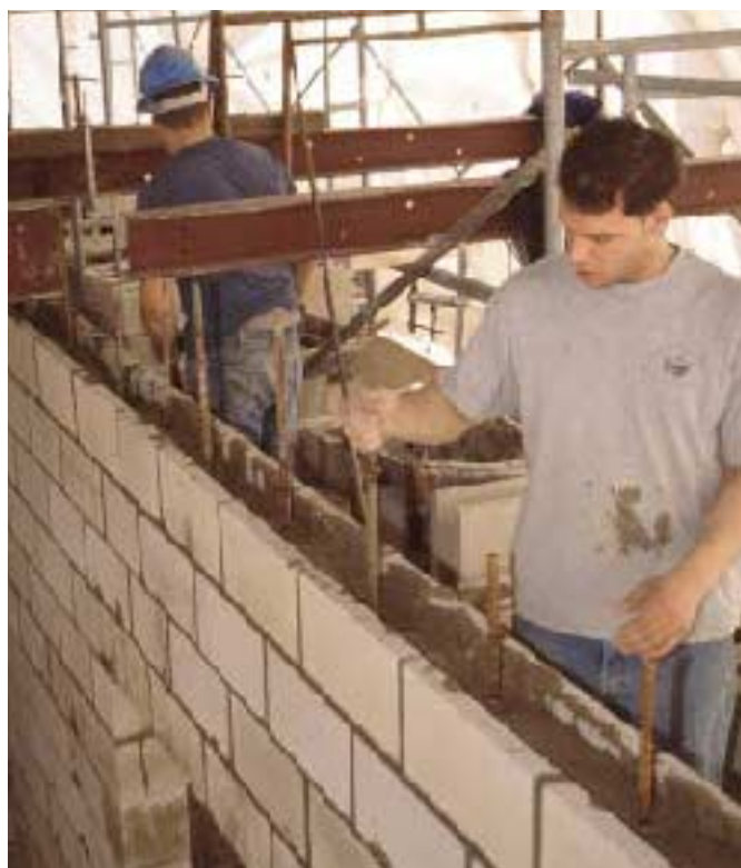
Figure 4. A simple overlap in the vertical rebar is all that's needed to provide continuity between lifts. The next course of block can then be lowered over the projecting rods without too much interference.
