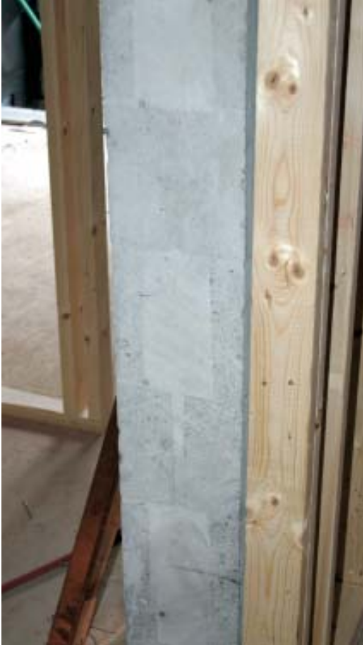
Figure 1. Completely grout-filled block cells are revealed in a cut made to widen an opening following a change order.
