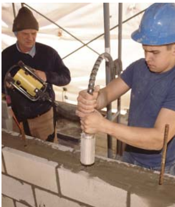
Figure 6. A rebar shaker quickly consolidates the grout in the cells, ensuring complete filling and embedment while saving time and labor.
