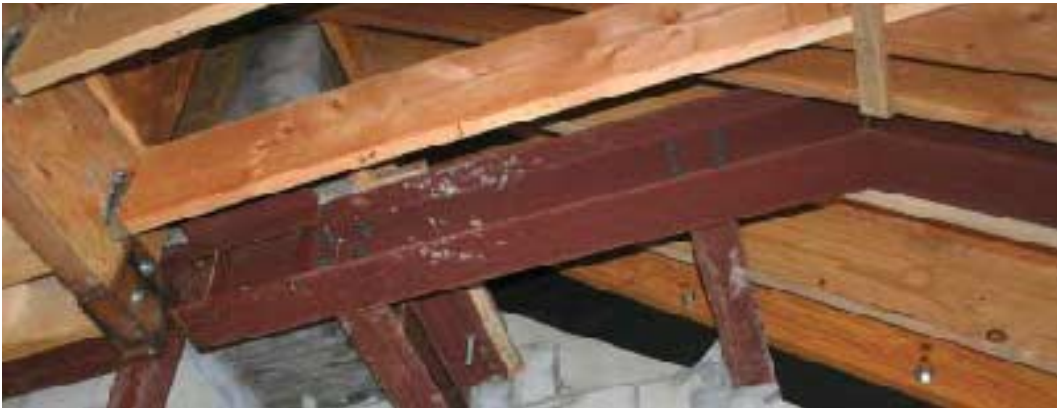
Figure 11. A steel frame, offset from the block wall but tied into it, supports the flue mass at each floor level.
