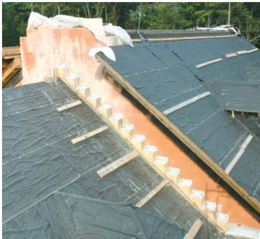
Figure 14. Galvanized steel lintels will support the exterior stone veneer above window openings. The lintel is bolted to the solidly grouted blockwork using epoxy-embedded anchor rods (right). Short lengths of steel lintel stairstep up the gables to support the finished stone veneer (below).
