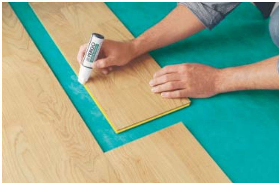
Figure 5. Glued joints are three times stronger than mechanical joints and can’t be forced open by flooring movement. Some glued products come with a preapplied adhesive that is activated when moistened. This prevents messy squeeze-out and ensures a continuous seal with just the right amount of adhesive.
