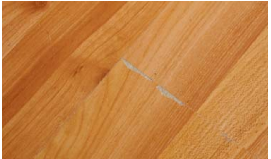
Figure 3. One problem with cheap laminate flooring products is fragile joints that can chip easily during installation.
