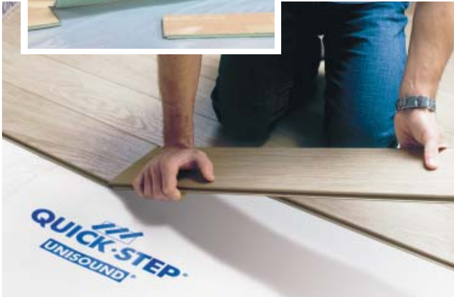
Figure 6. Rubberized foam underlayment puts a cushion beneath the floor and helps absorb minor bumps and deviations in the subfloor (below). It may be laid in sheet form or it may already be attached to the back of the flooring (inset).
