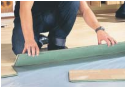
Figure 6. Rubberized foam underlayment puts a cushion beneath the floor and helps absorb minor bumps and deviations in the subfloor (below). It may be laid in sheet form or it may already be attached to the back of the flooring (inset).
