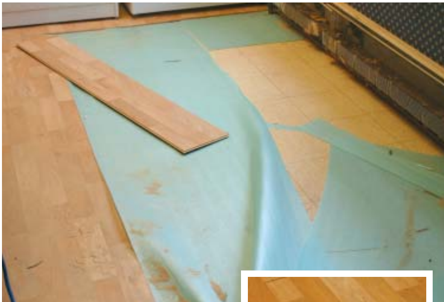
Figure 7. Two years after this floor was installed, obvious heaving appeared in the middle of the room. The problem was a pinhole leak in the hydronic baseboard heat that seeped underneath the floating floor to the lowest point. The flooring shrank after drying, leaving obvious gaps (inset). It had to be replaced (above).
