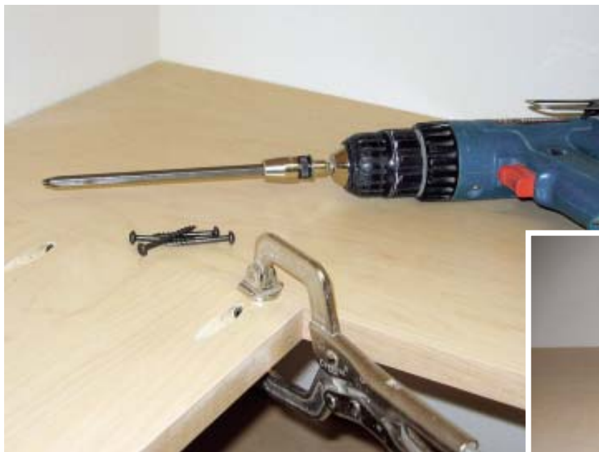
Figure 5. With pocket screws, the author can make a strong, tight joint with a minimal amount of labor. This shelf (above) is higher than eye level, so the screws go in from above. When the shelf is lower (right), the author hides the holes by installing the screws from below.
