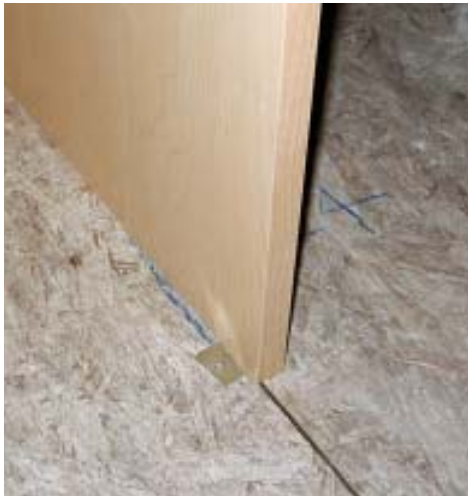
Figure 7. Thin enough to be covered by the finished flooring or by baseboard, small pieces of flashing nailed to the verticals hold the shelving in place.
