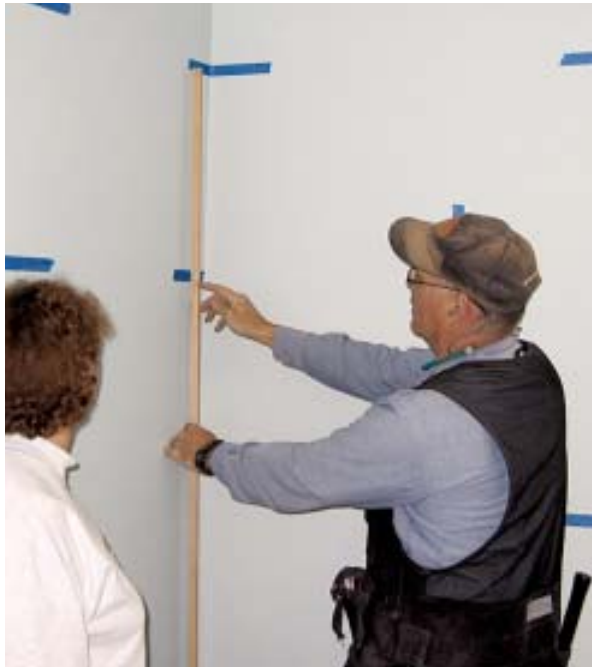
Figure 2. To help his clients visualize shelving options, the author uses a layout stick premarked with standard shelf measurements, and blue painter's tape to indicate potential shelf and support locations.
