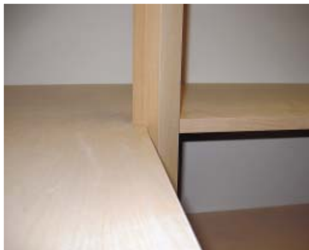
Figure 5. With pocket screws, the author can make a strong, tight joint with a minimal amount of labor. This shelf (above) is higher than eye level, so the screws go in from above. When the shelf is lower (right), the author hides the holes by installing the screws from below.
