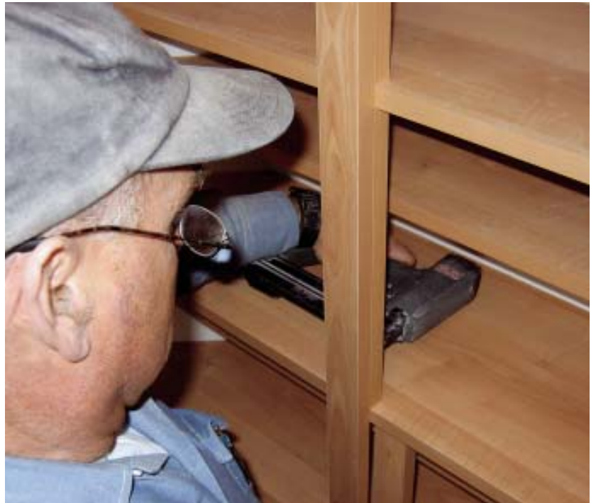
Figure 8. Short lengths of edged melamine help support the shelves. The author then overlays a second, continuous strip of melamine, fastening from behind to conceal nail holes.
