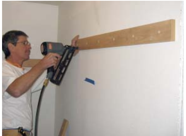
Figure 3. Drilled to accept Shaker-style clothes pegs, this cleat was edged by the cabinetmaker in the shop and then cut to fit on site; only the ends were edged in the field.
