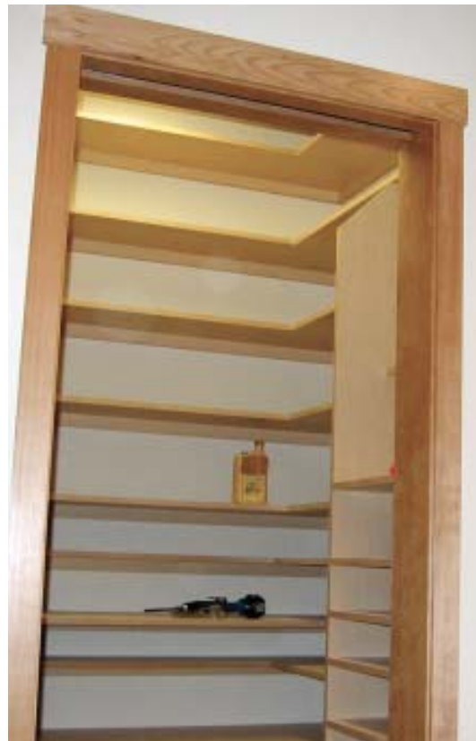
Figure 1. The author buys the entire closet package from a cabinetmaker who rips melamine into shelves and cleats before banding them with a matching edge (above). This nearly eliminates ripping and edging material in the field and allows customers to get highly customized shelving in virtually any color or pattern they want.
