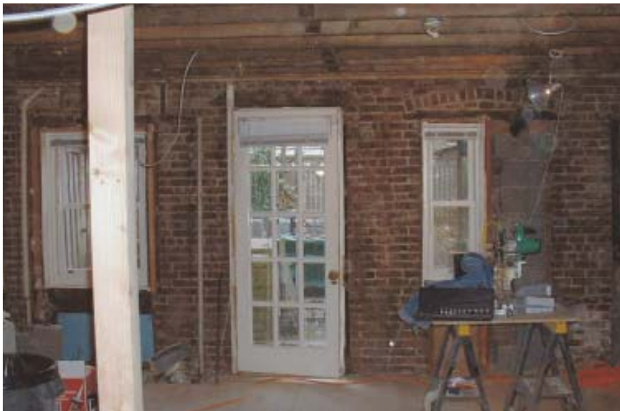
Figure 1. As the centerpiece of an extensive garden-level remodel, the new four-panel glass door would open up the ground level to the backyard, filling the dark room with natural light. First, though, a 12-foot-wide rough opening needed to be cut in the solid brick exterior wall of the Hoboken, N.J., home.
