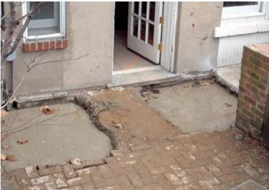
Figure 4. To prevent the braces from kicking out from the wall under load, the footings were buried below grade. The author used a transit to make sure the poured footings were level with each other.
