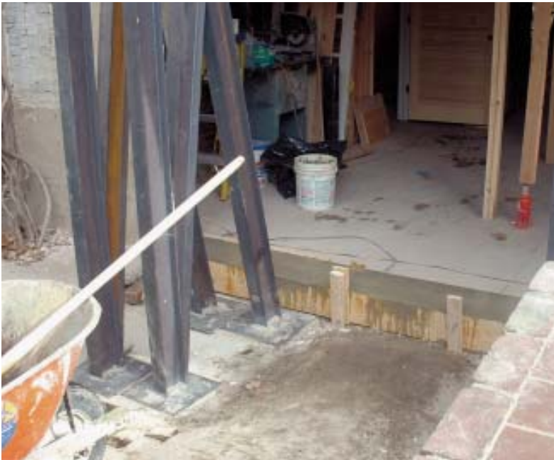
Figure 7. Formed on top of the broken-out foundation wall, the newly poured threshold offered a smooth, level reference point for laying out the rough opening. The brick side walls shown in the photo at right would receive a smooth mortar cap before installation of the new door.
