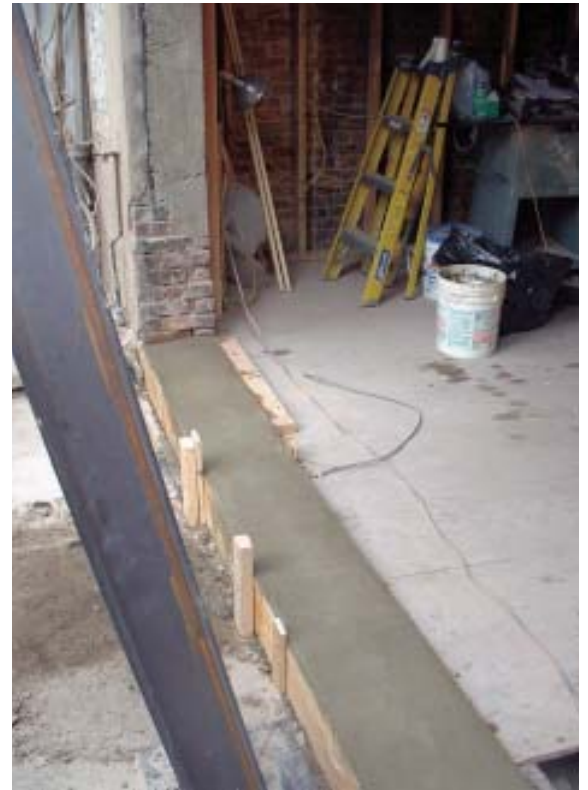
Figure 7. Formed on top of the broken-out foundation wall, the newly poured threshold offered a smooth, level reference point for laying out the rough opening. The brick side walls shown in the photo at right would receive a smooth mortar cap before installation of the new door.
