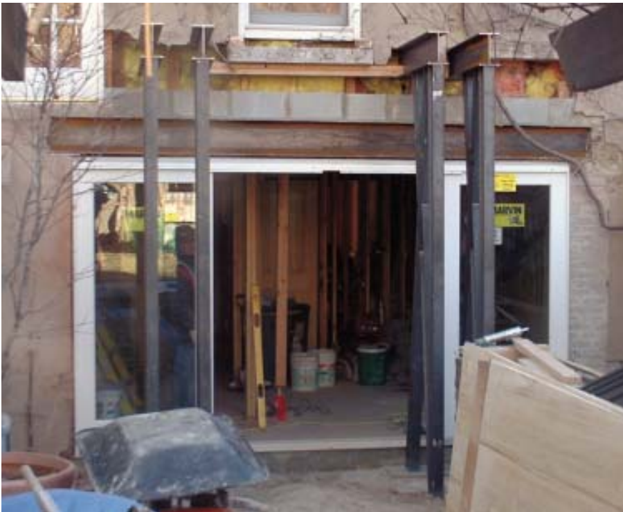
Figure 8. A pair of 5 1/2-by-10-inch steel beams supported the masonry above the new door opening. The author chose to install the door before removing the braces, making it easier to secure the site during construction.
