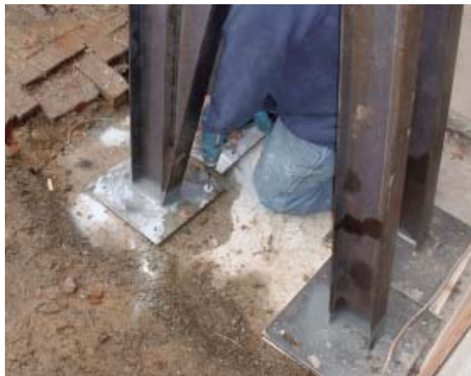
Figure 6. Once the braces were maneuvered into position, the crew shimmed them (above) and bolted them securely to the concrete footings with wedge bolts (right).
