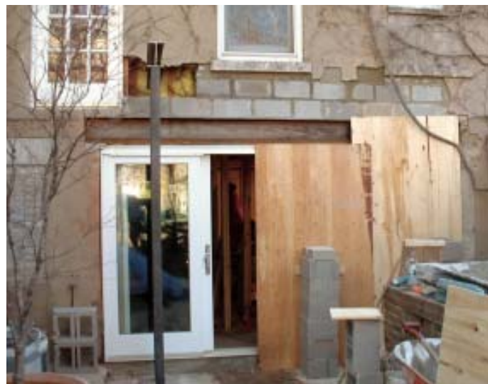
Figure 9. Because the masonry wall has a stucco finish, economical 12-inch block instead of brick was used to fill in above the new steel header (above left). The author's crew made sure each section of wall was well supported with block before removing the braces, one at a time (above). Mortar dye added to the stucco matches the new work to the existing wall (left).
