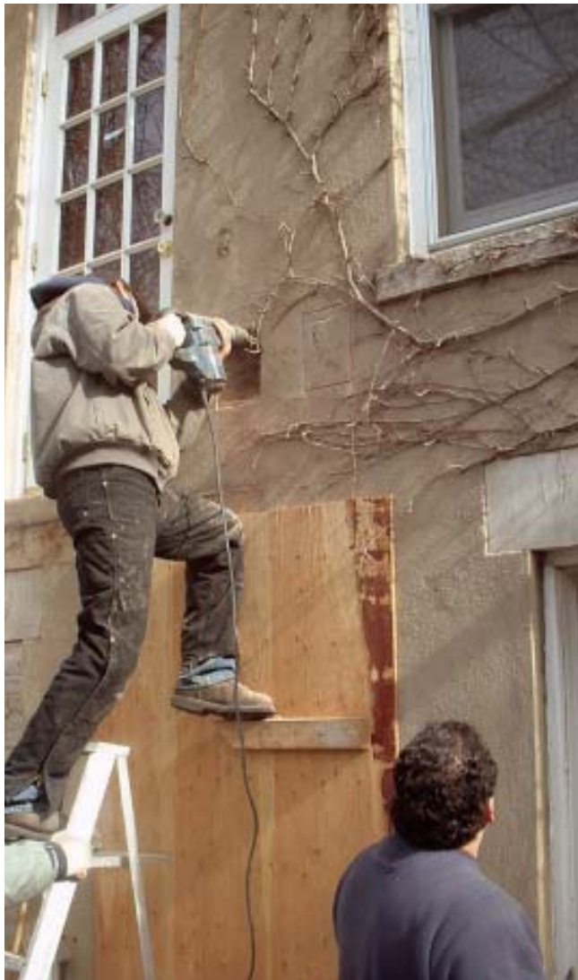
Figure 5. After placing the braces on their footings and marking their positions on the wall, the author's crew cut 8-inch-deep pockets into the 12-inch-thick masonry wall for the upper shelf of each brace.
