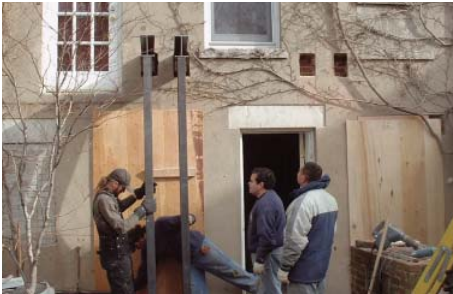
Figure 6. Once the braces were maneuvered into position, the crew shimmed them (above) and bolted them securely to the concrete footings with wedge bolts (right).
