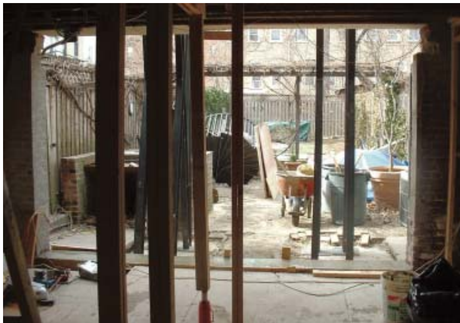
Figure 1. As the centerpiece of an extensive garden-level remodel, the new four-panel glass door would open up the ground level to the backyard, filling the dark room with natural light. First, though, a 12-foot-wide rough opening needed to be cut in the solid brick exterior wall of the Hoboken, N.J., home.
