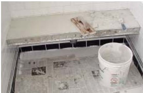
Figure 4. Once the frame was installed, the author filled the tray with deck mud and screeded off the excess to create a level setting bed for the tile. After setting and grouting the tile, he sealed the perimeter of the bench with a color-matched caulk.
