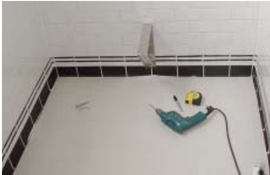
Figure 2. Bench spans of greater than 36 inches require a triangular corbel. To simplify tile installation, the author filled the corbel with mortar and tiled it before installing the bench top.
