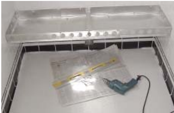
Figure 3. Measuring 14½ inches wide by 3½ inches deep, the bench's aluminum frame adjusts from 33½ to 62 inches long. While it can be attached to walls with hollow wall anchors and adhesive caulk, the author used lag bolts that fasten to blocking installed during framing.
