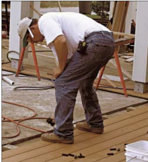
FIGURE 5. Borden relies on hidden deck fasteners when zoning requirements allow. He typically uses Eb-Ty “biscuits” (top left) that get installed in a kerf cut in the edge of a board with a plate joiner, or Tiger Claw fasteners (top right). The Tiger Claw install faster in hardwood, but they’re difficult to pound into the edge of composite decking. For composites, it’s better to use the decking manufacturer’s proprietary fasteners, such as those made by Eb-Ty for CorrectDeck (above).
