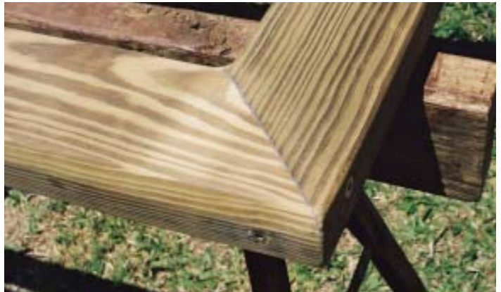
Figure 8. The gate's mitered corners are assembled with 4-inch stainless-steel screws, Lamello K-20 plastic biscuits, and two-part epoxy. Ulmia miter clamps from Garrett Wade (800/221-2942, www.garrettwade.com ) hold the assembly together while the epoxy sets. The author prefers an intermediate rail to the more traditional diagonal brace because it matches the rest of the fence and provides space to mount the latch.
