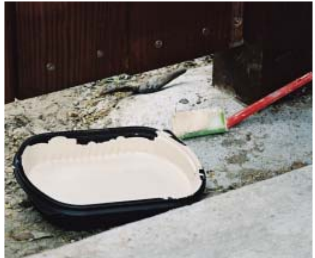
Figure 9. Designed primarily for industrial applications, two-part coatings have better adhesion and a higher percentage of solids than conventional one-part paints. The author uses them to prevent water from entering vulnerable end grain (left and below left). Bending the handle on a foam brush makes coating the bottom of fence boards easier (below).
