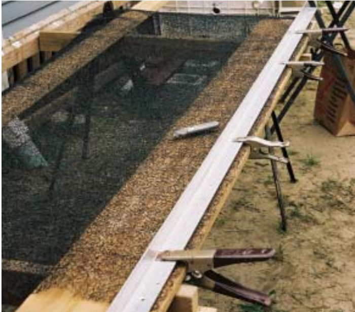
Figure 6. A 1/8-inch gap behind the fence boards — created by fastening Enkamat to the rails with stainless-steel staples — keeps water from being trapped (left). Similar gaps are left where the horizontal rails meet the posts. The author fastened the L-shaped brackets securing the rails with 1½-inch-long #8 pan-head screws and oriented them so that the brackets are hidden behind the fence boards (above). Some rail ends were cut on a slight angle or bevel to match warped or twisted posts.
