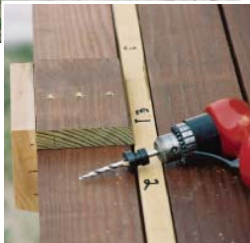
Figure 5. The screw pattern on the first full-sized fence board is laid out by hand, but then it becomes a jig for the rest of the boards when the author screws registration blocks on one end and one side (above). Smaller boards next to the post get their own jig. A WL Fuller Co. tapered bit (401/467-2900, www.wlfuller.com ) does the drilling and counter-sinking in one step (right).
