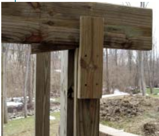
Figure 7. The simplest tool is also one of the best. A small wedge cut from scrap can very accurately raise or lower a heavy work-piece into place. Here a wedge is used along with the author's header-board holder to bring the header flush to the leveled top of a post.
