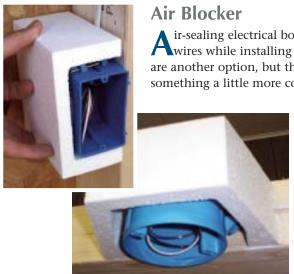
Air-sealing electrical boxes is tough to do. You can use caulking or duct seal, but flexing the wires while installing the device is likely to ruin the seal. Special work boxes with gaskets are another option, but they're expensive and I'm betting that your electrician would prefer something a little more conventional. After struggling with this problem for years, Joel Ander-
