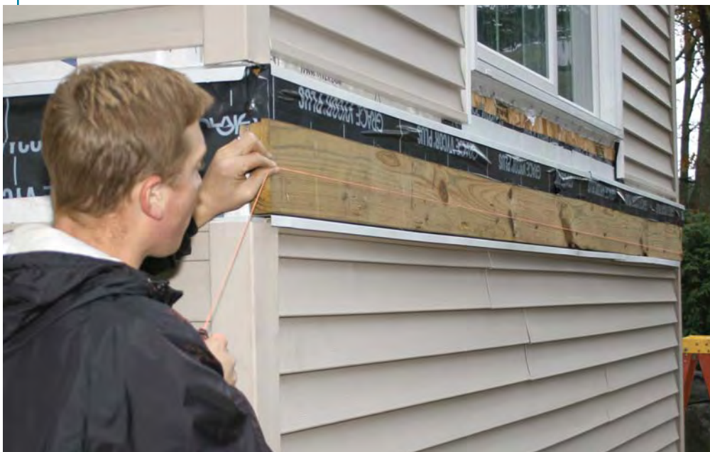
Figure 3. Houses aren't always straight, so the author checks the ledger with a string. Variations greater than \frac{1}{4} inch mean that the joists will have to be custom cut.
