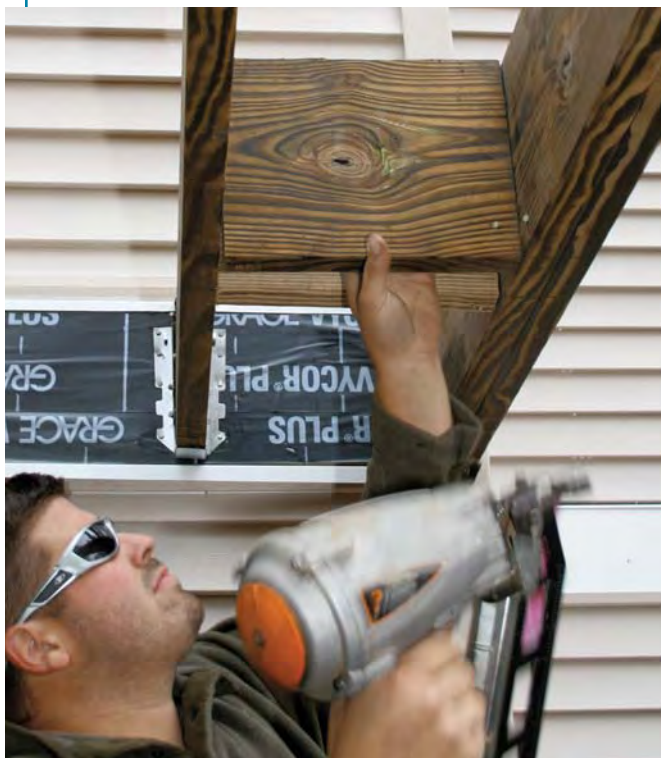
Figure 12. The last step in framing is installing blocking for items such as benches, decking patterns, or planters.
