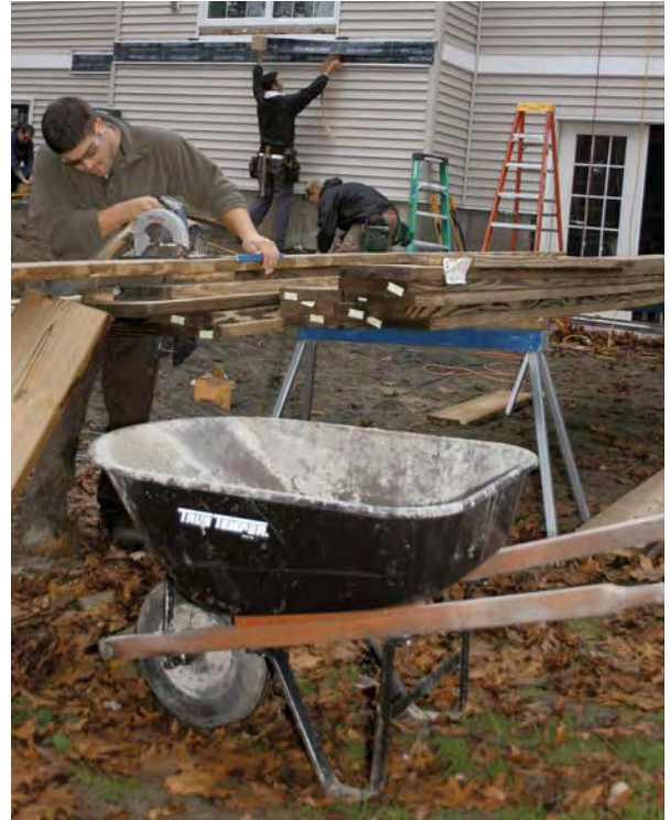
Figure 2. Setting up a wheelbarrow or garbage can for scraps at the cutting station is an easy and fast way to keep the site cleaner.
