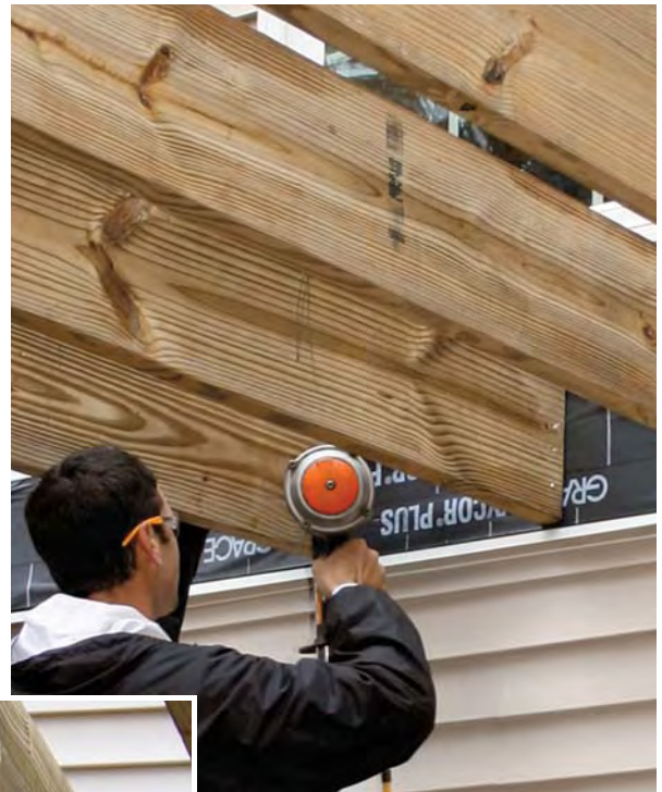
Figure 9. Resting the joists on the girder, one carpenter toenails them in place (above). A second crew member follows behind, using a metal-connector nailer to fasten the joist hangers (left).
