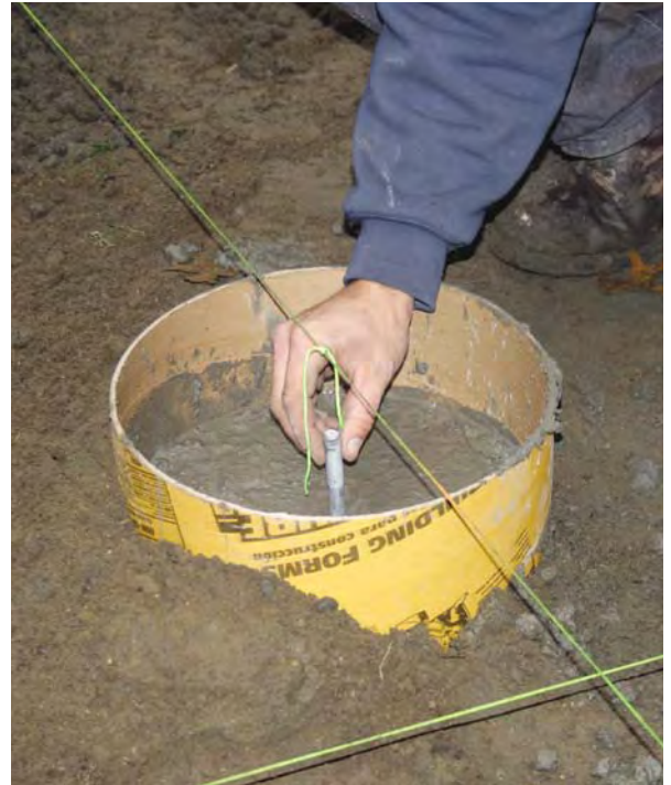
Figure 7. Precise placement of anchor bolts speeds locating the post bases.
