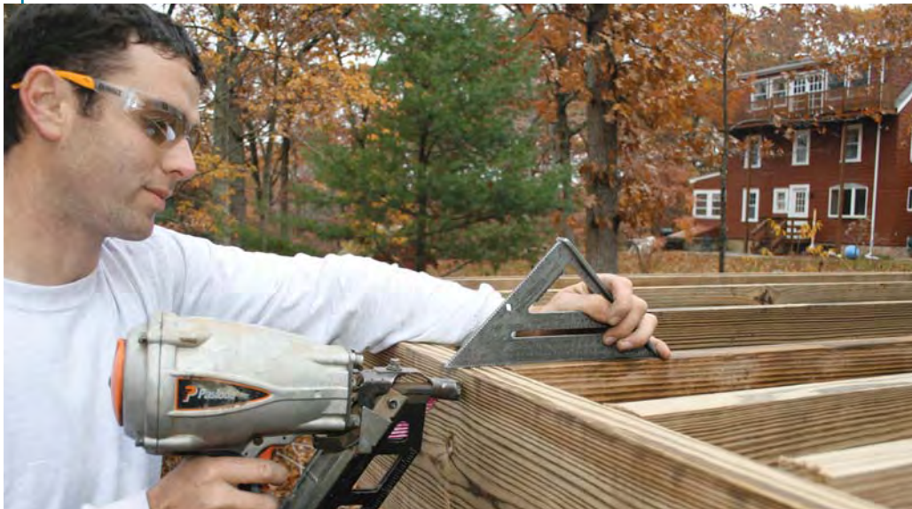
Figure 10. Before being attached to the beam, the joists are leveled with and nailed to the rim joist. Shims are added between the joists and the beam if needed; then the pre-installed hurricane ties are nailed to the joists.
