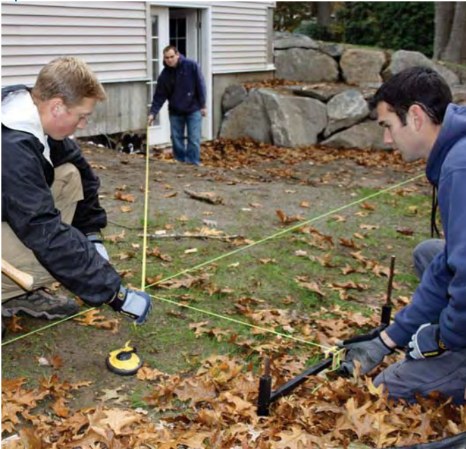
Figure 5. While one crew member starts cutting, others lay out the footings using a precalculated length for the diagonal measurement.
