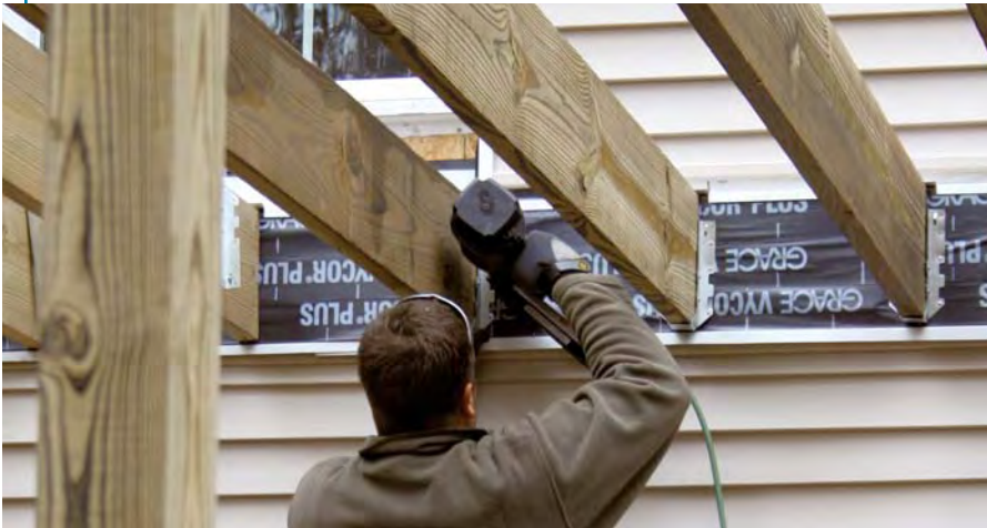
Figure 9. Resting the joists on the girder, one carpenter toenails them in place (above). A second crew member follows behind, using a metal-connector nailer to fasten the joist hangers (left).
