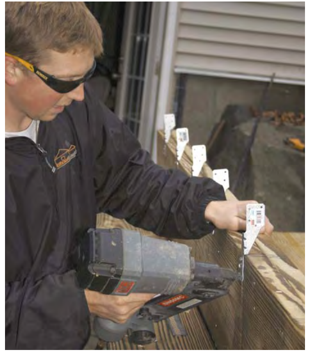
Figure 4. The person assigned to the cut station also assembles the beams, going so far as to lay them out and nail on the hurricane ties.
