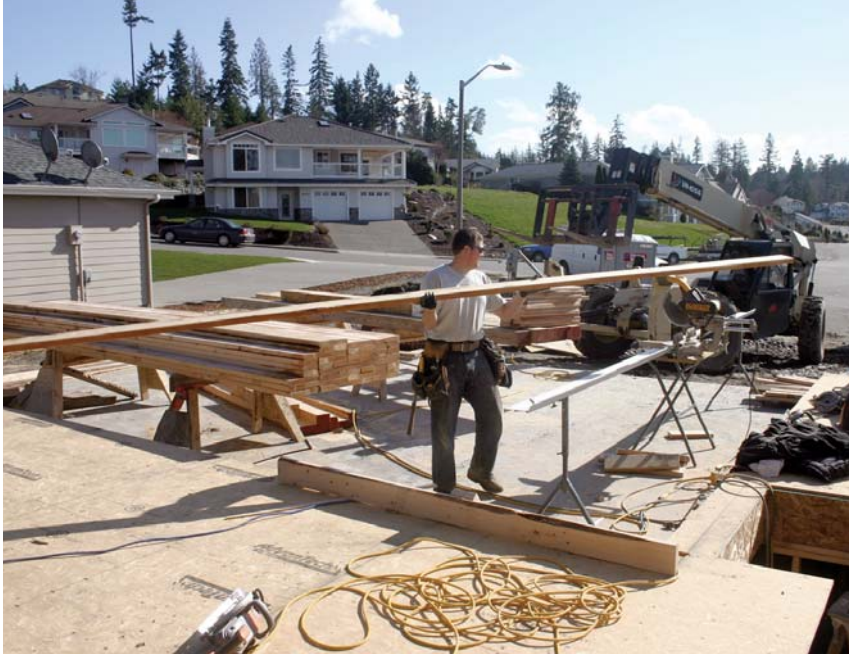
Figure 1. The crew positions a pile of 20-foot 2x6s within easy reach of both the sawyer — who uses them to cut window packages and blocking — and the layout person, who uses them to make plates.
