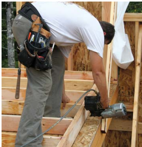
Figure 5. Working as a team, one carpenter packs material and crowns studs (above) while the other tacks the bottom plate to the deck (far right) and nails walls together (right).
