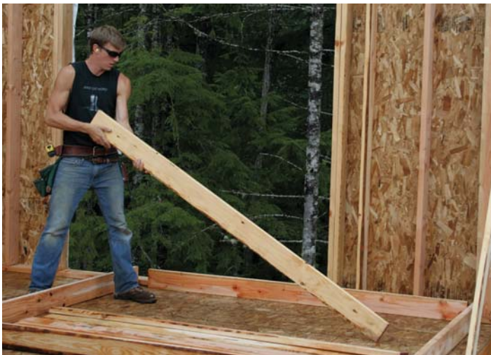
Figure 5. Working as a team, one carpenter packs material and crowns studs (above) while the other tacks the bottom plate to the deck (far right) and nails walls together (right).
