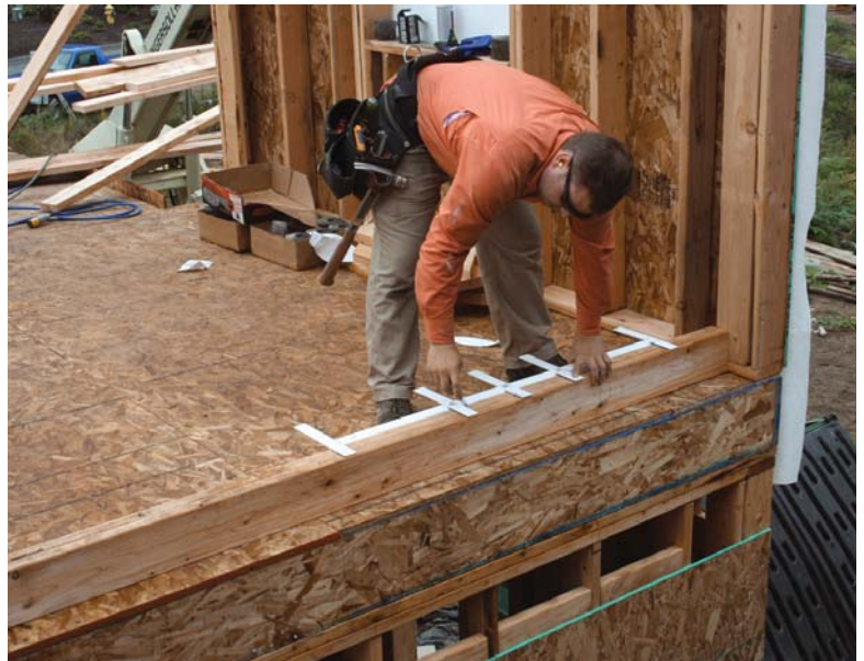
Figure 2. The author cuts exterior wall plates two at a time with a Big Foot saw (left). After marking the location of door and window openings, he uses a layout stick to space the studs (above).
