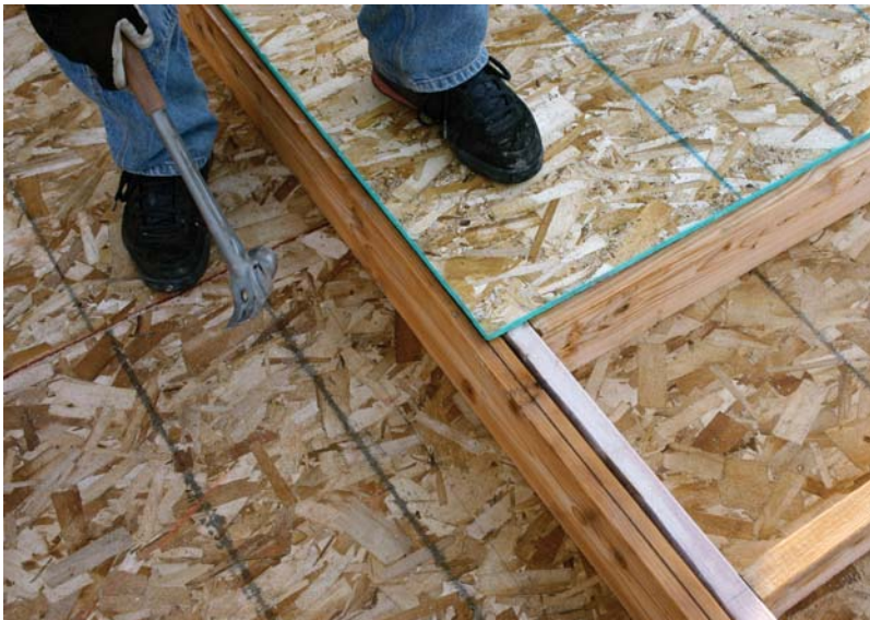
Figure 7. Sheathing will run off layout if it's nailed flush to a plate that isn't straight. To avoid this problem, the author aligns sheathing with a snapped line \frac{3}{4} inch down from the top of the double top plate (above). After nailing it off, he cuts out openings with a router (right).
