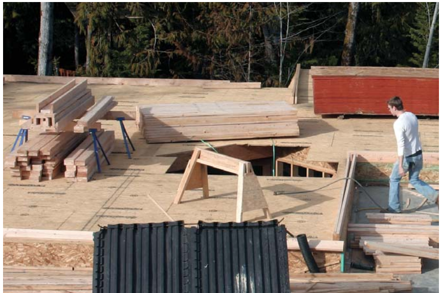
Figure 4. A carpenter cuts trimmers from a pile of studs in the center of the deck (left). The finished corners and king stud-trimmer combos (above) are stacked next to the stud pile — close to where they'll be needed when the walls are assembled.
