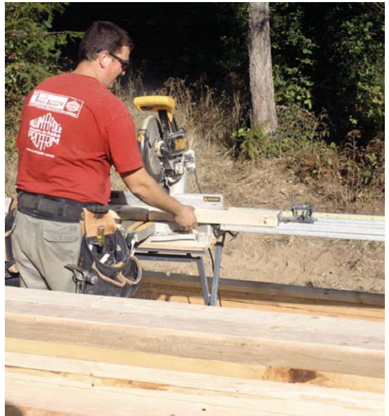
Figure 3. It's faster to cut short pieces with a miter saw and stop than to measure and mark individual pieces and then cut them with a circular saw.
