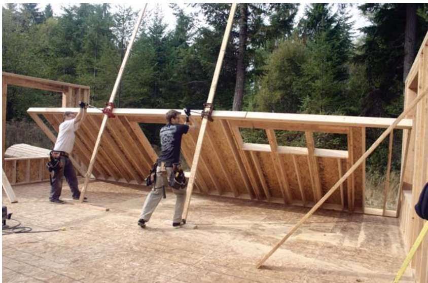
Figure 8. An all-terrain forklift can stand walls too heavy for a small crew to lift (top). When there isn't sufficient access for the machine, the author's crew uses wall jacks (above).
