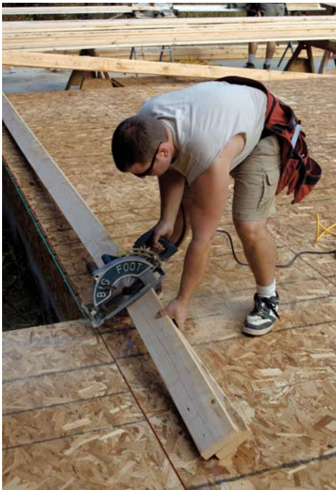
Figure 2. The author cuts exterior wall plates two at a time with a Big Foot saw (left). After marking the location of door and window openings, he uses a layout stick to space the studs (above).
