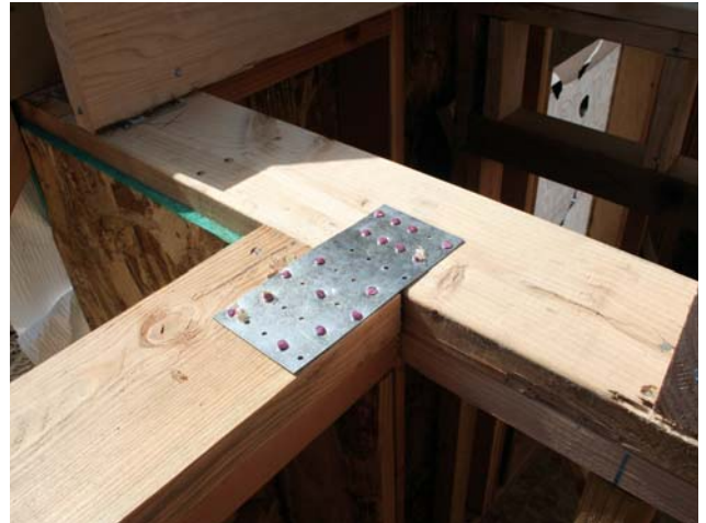
Figure 6. Instead of lapping double top plates, the author's crew installs tie plates at the ends of walls (above left) and uses them to hold the corners together (above). This method is permitted by the IRC, provided the plate is at least 3 inches by 6 inches by .036 inch thick and fastened on either side with a minimum of six 8-penny nails.
