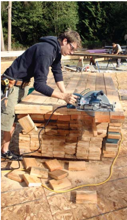
Figure 4. A carpenter cuts trimmers from a pile of studs in the center of the deck (left). The finished corners and king stud-trimmer combos (above) are stacked next to the stud pile — close to where they'll be needed when the walls are assembled.
