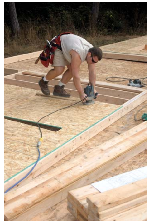
Figure 7. Sheathing will run off layout if it's nailed flush to a plate that isn't straight. To avoid this problem, the author aligns sheathing with a snapped line \frac{3}{4} inch down from the top of the double top plate (above). After nailing it off, he cuts out openings with a router (right).
