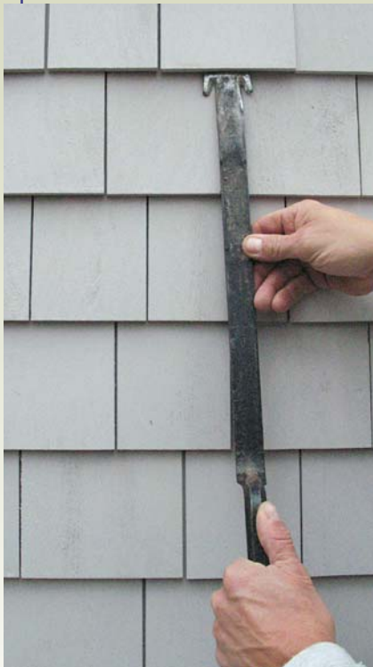
Figure 7. A slate ripper slips between courses of siding, where its J-shaped hooks grab the nail shanks (above left). A couple of downward hammer blows will either cut or pull the nails (above right).
