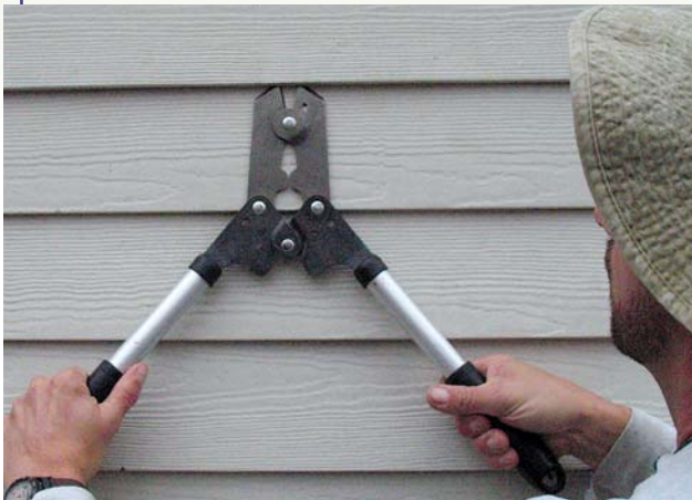
Figure 11. Thin-bladed nail cutters slide under a course of siding to snip the fasteners.
