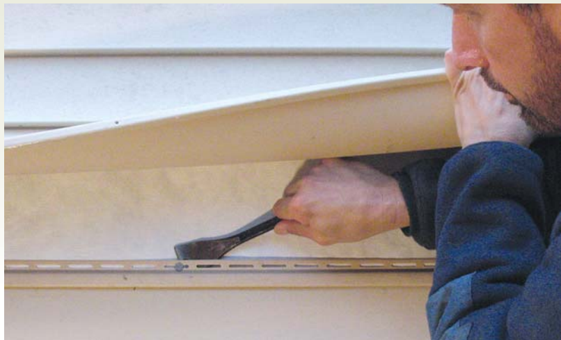
Figure 15. With the upper piece exposed, vinyl siding's fasteners are easily accessed.
