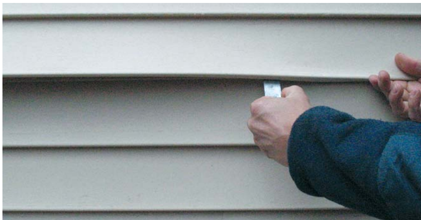
Figure 14. A J-shaped zip-lock tool (above) grabs the bottom lip of vinyl siding, disengaging it from the course below (right).
