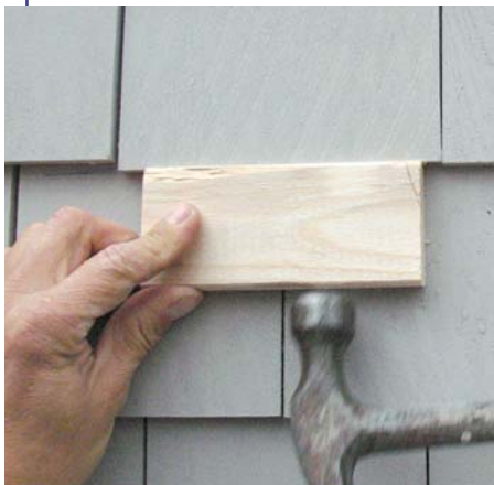
Figure 9. To blind-nail a replacement shingle, hold it slightly below its intended location and nail it just below the butt line of the course above. A few taps with a block and a hammer drive the shingle into place, bending the nails mostly out of sight at the same time.
