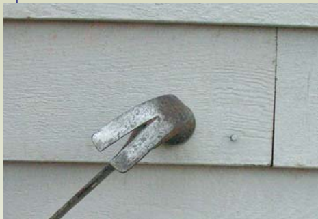
Figure 3. A gentle tap forces the clapboard down, leaving the nail head proud of the surface so it can be gripped with wire nippers.
