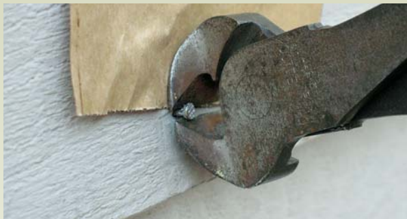
Figure 3. A gentle tap forces the clapboard down, leaving the nail head proud of the surface so it can be gripped with wire nippers.
