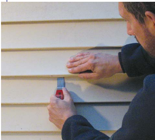
Figure 16. The zip-lock tool pulls the lip back down, and hand pressure following behind reseats the upper vinyl panel in the lower.
