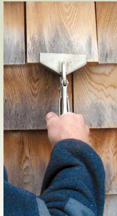
Figure 8. Wide-jawed locking pliers exert enough clamping pressure to allow a shingle to be wiggled free of its nails.
