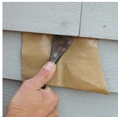
Figure 2. Careful prying near the face nail often lifts both the siding and the nail.
