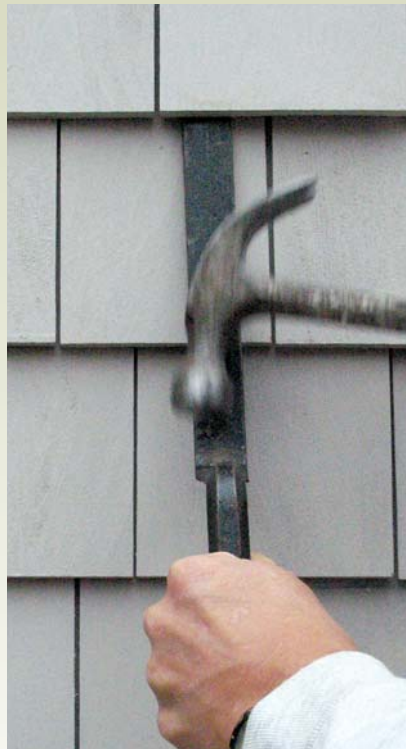
Figure 7. A slate ripper slips between courses of siding, where its J-shaped hooks grab the nail shanks (above left). A couple of downward hammer blows will either cut or pull the nails (above right).
