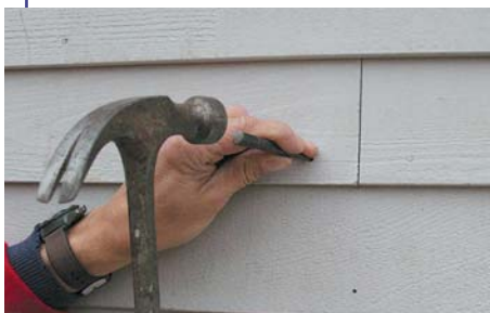
Figure 5. Driving nails through the siding with a nail set leaves large holes. Reinstallation is still possible — just use nails with larger heads in the same holes.
