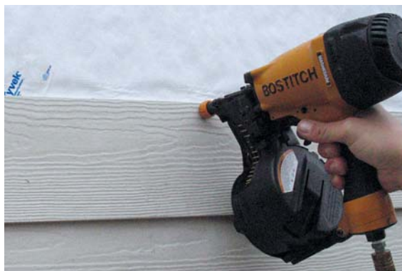
Figure 12. Fiber-cement siding is best installed with a nail gun. Otherwise, nail holes must be predrilled. In either case, set the nails flush with the face of the siding and no deeper.
