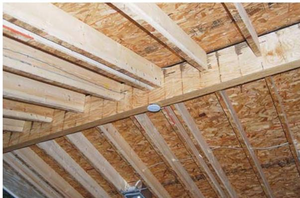
Figure 11. Cathedral ceilings rely on stout ridge beams, rather than a rafter-joint triangle, to prevent sagging.
