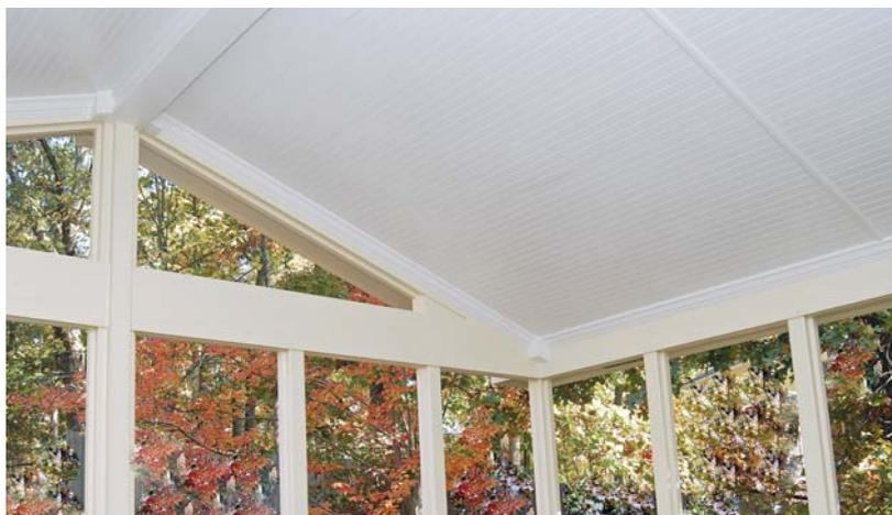
**Figure 13. Painted beadboard ceilings provide a great finished look and brighten the space more than stained wood.**
