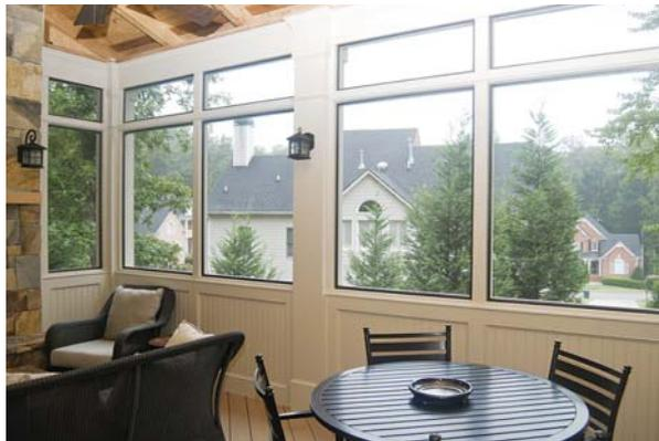
**Figure 7. Knee-walls provide guards, privacy, and a place for electrical outlets.**
