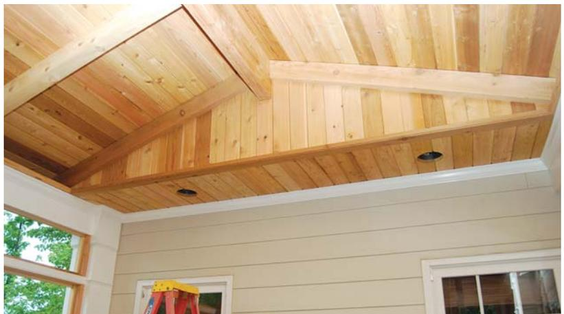
**Figure 2.** Covering a house's second-story cantilever with the same material that's on the porch ceiling helps to blend it in.
