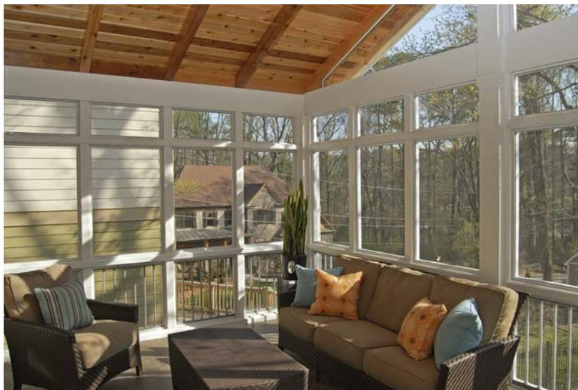
**Figure 8. Timber rafters that stack atop the posts provide a clear load path. Tongue-and-groove 2-bys above provide both a finished ceiling and a roof deck.**
