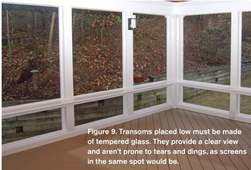
Figure 9. Transoms placed low must be made of tempered glass. They provide a clear view and aren't prone to tears and dings, as screens in the same spot would be.
