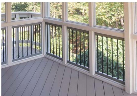
**Figure 6. Elevated porches — even when screened — require guards to prevent falls.**
