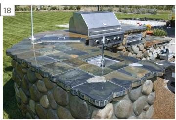
edge. I then used a series of diamond polishing discs (up to 1,500 grit) to give the edge a comfortable, easy-to-clean honed finish. I did this before grouting, to prevent scratching.
