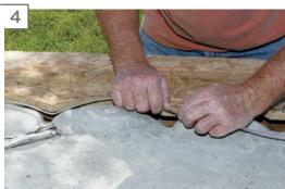
jigsaw, then screwed the OSB strips to the 2x4s. This gave me a ledge flush with the top of the base and close to the rocks beneath. I then drew a line freehand to mark the edge of the top, allowing for about a  $2^{1}/2$ -inch overhang beyond the face of the rock veneer.
