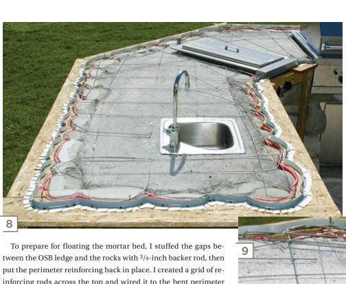
inforcing rods across the top and wired it to the bent perimeter rods (8). To prevent the forms and screeds from spreading while I compacted the mortar bed, I also used tie wire to draw the opposing sides together, running it beneath the reinforcing rods (9).
