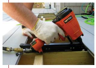
nd slow, my standard methcallation had been to place a groove on the deck board, e a small screw into the clip and joist using either a cordless drill or an impact driver. That is, until recently, when Tiger Claw, a maker of hidden deck fasteners, introduced the TC-Gun.
