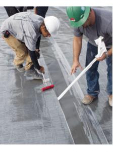
must go on before the concrete is poured. *MiraPly* self-adhering blind-side waterproofing can make a difficult job just a bit easier. According to the maker, the thermoplastic polyolefin membrane is coated with a butyl adhesive that forms a permanent bond with the poured concrete. It comes in two formulations: one for vertical applications and another for horizontal (underslab) applications. The manufacturer declined to provide pricing.
