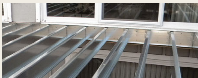
Figure 5. Attach the steel ledger to the house as you would a wood one, with \frac{1}{2} -inch lag bolts and standard flashing details.
