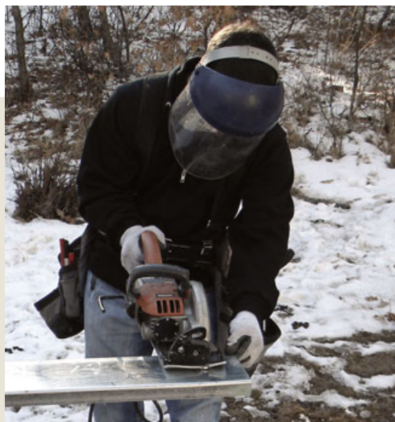
Figure 4. Full face and hearing protection and a special blade for ferrous metals are needed to cut steel joists.
