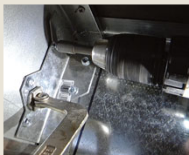
Figure 3. Use a locking C-clamp to position steel members and predrill for screws.
