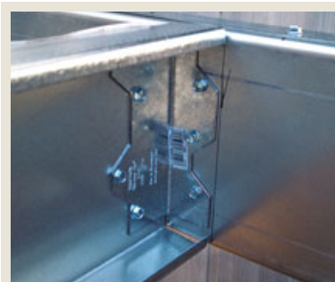
Figure 2. Standard framing hardware and galvanized sheet-metal screws join the members.
