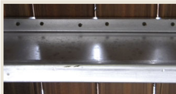
Figure 15. Decking can be fastened to steel joists with screws from below.
