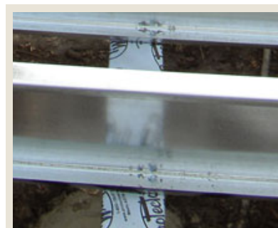
Figure 8. Protect the tops of beams from water with a layer of flashing membrane.
