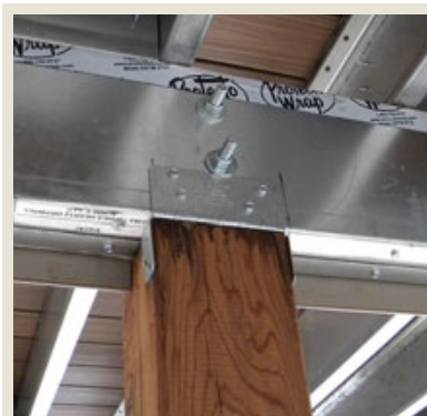
Figure 11. Wood posts can be joined to steel beams with regular hardware.
