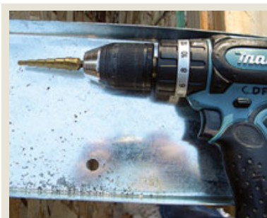
Figure 6. Predrill the ledger for the \frac{1}{2} -inch lags using a step drill.
