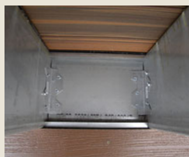
Figure 9. Blocking is required between joists where they bear on the beam.
