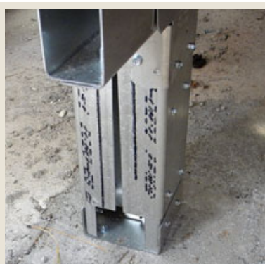
Figure 12. A short piece of track bolted to the footing serves as the post base for a steel post.
