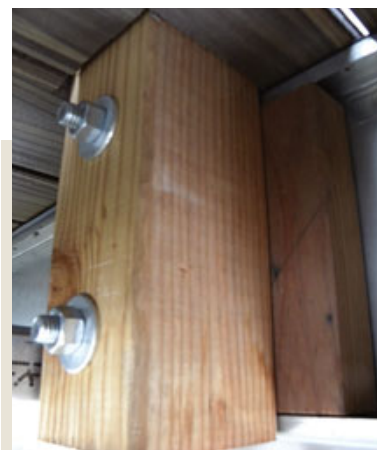
Figure 13. Attach newel posts to steel framing with two 1/2-inch bolts. If the posts are pressure treated, separate them from the steel with flashing membrane.
