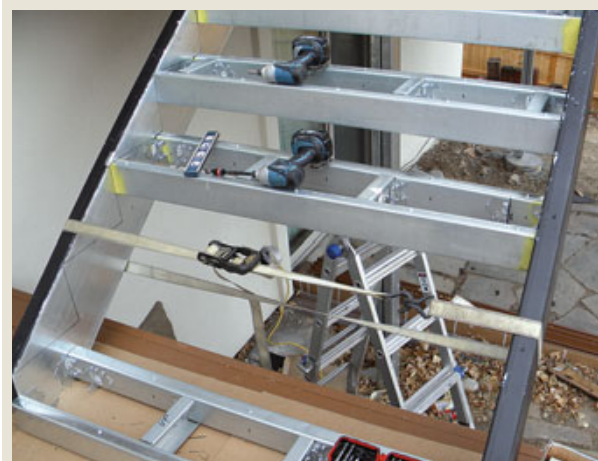
Figure 14. Stairs can be built from steel, but the process is time-consuming. Because of this, the author generally uses wood stringers.
