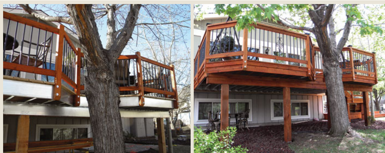
Figure 1. Once wrapped in finish material, lightweight steel-framed decks look pretty much like any other deck.
