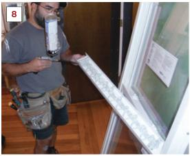
which fits over the top of the frame and slides up to fill the space between the top of the window frame and the head jamb.
