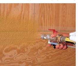
based sheathing. The maker claims that the coating is compatible with all common types of siding and exterior finishes; that it qualifies as both an air and a moisture barrier; and that it won't rip or blow off. Installation costs range from \$1 to \$1.20 per square foot.
