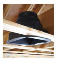
sheet-metal diffusers. Installers should appreciate the product's versatility: Each of the available sizes (6x6, 8x8, and 10x10) has a stepped collar that lets it connect to three different diameters of flexible ductwork.
