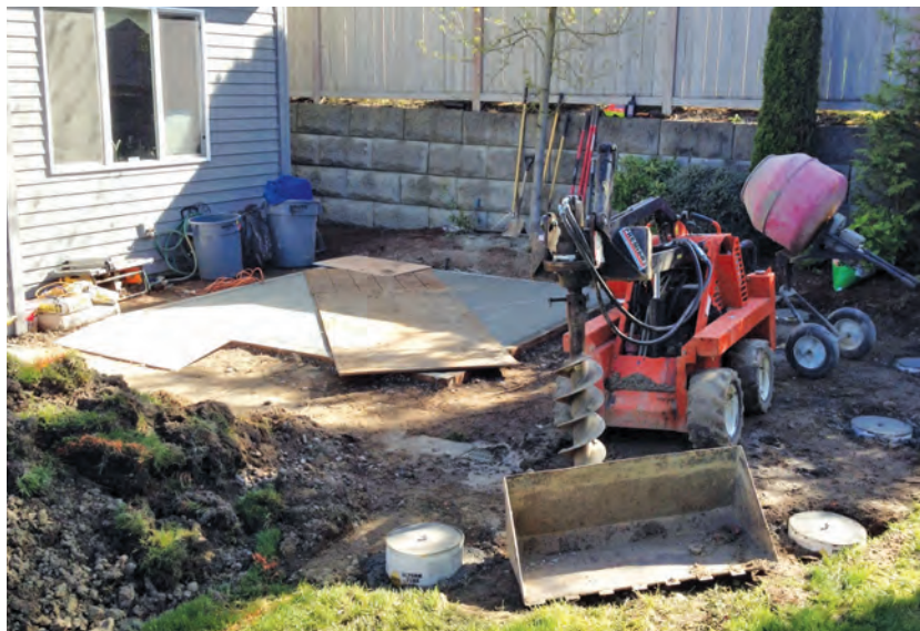
Figure 1. Ground-level hot tubs are typically supported by a concrete slab, which should be formed and poured at the same time as the deck footings.
