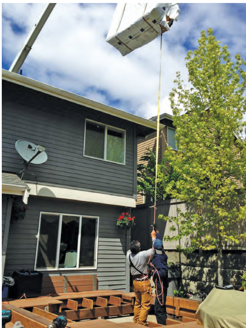
Figure 3. Suppliers are usually responsible for delivering and placing the hot tub, but it's up to the deck builder to make sure the supporting structure is sized correctly and that necessary utilities are in place prior to delivery (top). It sometimes takes a little extra time and ingenuity to deliver a large hot tub to its final destination. When hiring a crane, be sure the hot tub doesn't exceed weight limitations, and that the crane has adequate reach (above).
