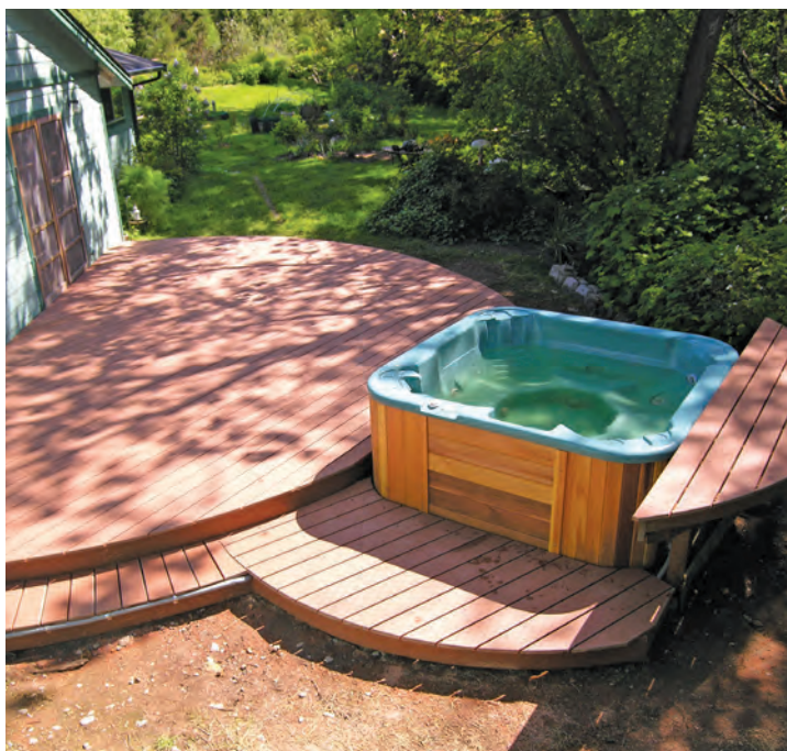
Figure 7. A spa table is a handy hot-tub option that can provide a place to sit and dangle feet in the water, or to set a drink. The table should be designed so that it doesn't block access to the spa's plumbing.
