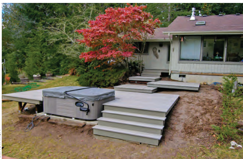
Figure 5. A flush-mounted hot tub (above) can present safety issues. When the edge of the tub is at seat level, access is safer and easier (left).
