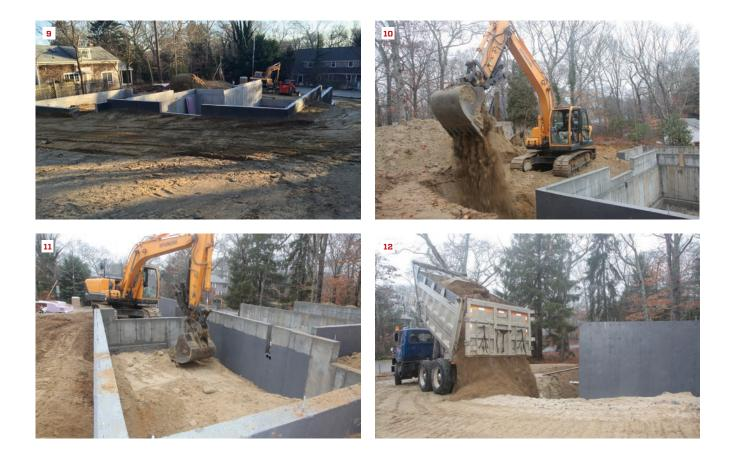
level as the grade at the driveway and garage floor. On two sides of the house, the foundation walls extend almost two feet above the shelf to allow the grade next to the foundation to be higher than the floor and then slope away from the house properly (9).
