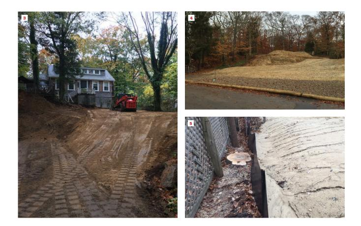
site is stripped and stockpiled safely on the lot for use during final grading. But because this site was so overgrown and littered with surface rocks, separating out the loam was not worth the effort.
