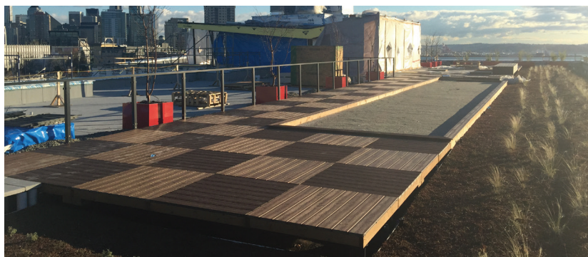
Figure 5. With the aluminum railing sections slipped down over the stanchions, the deck is nearing completion. Yet to be installed is the fascia, which will wrap around the entire deck to box it in.
