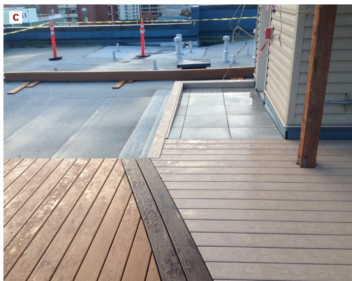
Figure 1. Bison Versadjust pedestals (A) were used to support the large-format stone pavers on this sloped access ramp (B, C). The adjustable pedestals can also support conventional wood framing, as well as the 4x4 grids shown in this article.
