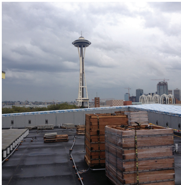
Figure 2. To avoid damage to the roofing, the author's crew prefabricated modular 4-by-4-foot deck grids on the ground, stacked them on pallets, and lifted them up to the rooftop with a crane.
