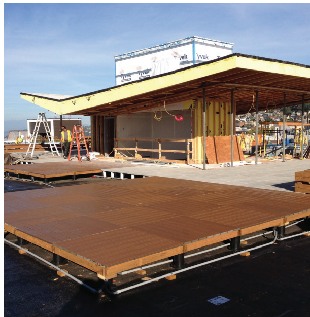
Figure 3. Once installed on top of the pedestals, the grids were fastened together with long structural screws.
