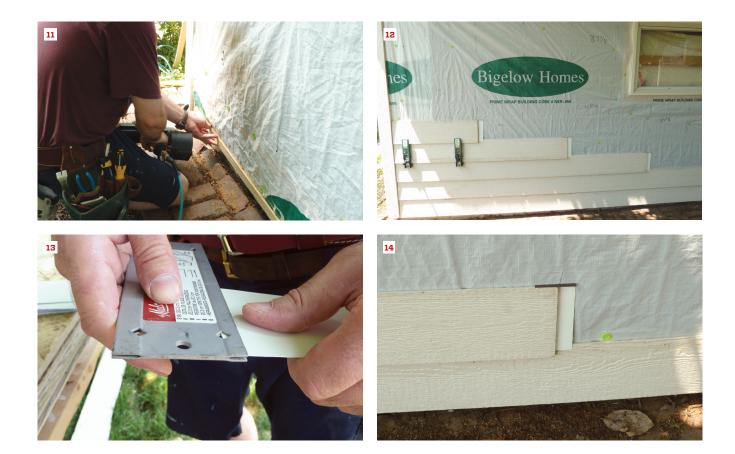
with a chalk line or a straightedge. These marks represent the *bot-tom* edge of each course and will be impossible to see as the siding is installed. So after the reference lines are drawn or snapped, I transfer them onto the edge of the trim where they can be read as the siding is installed.
