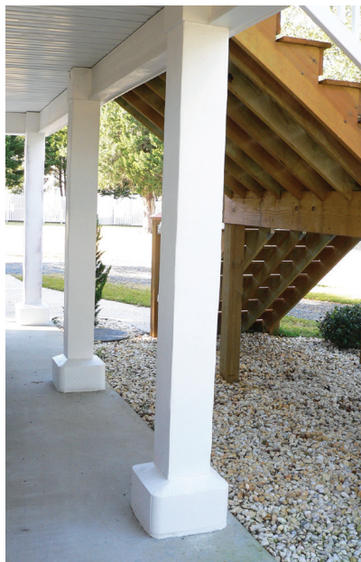
Figure 8. Because the steel columns supporting the deck at ground level are in a flood plain, the author wrapped them with masonry block finished with stucco.
