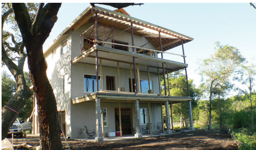
Figure 5. Shoring must be installed to support the panels during the pour, and it's left in place while the concrete cures. Here, the pour stops have been removed from around the perimeter, showing the 1 1/2-inch formed overlap that allows for a drip edge over the trim that will be fastened to the steel girders.
