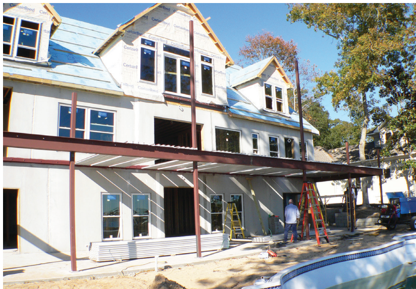
Figure 2. Around the perimeter of the deck, the I-beams that support the panels are welded to 4x4 steel columns.
