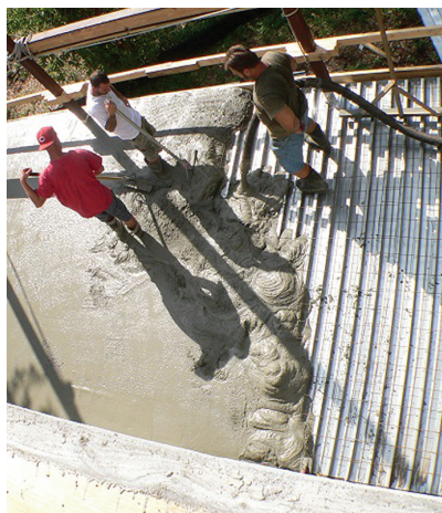
Figure 6. Concrete for the actual pour must be delivered with a pump truck.
