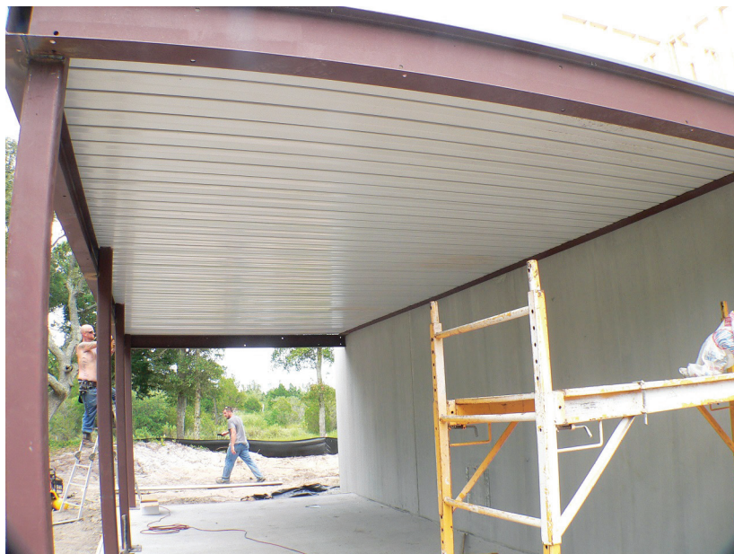
Figure 7. The porch slab cures for about 28 days, after which the shoring can be removed, and finish materials applied to the steel frame.
