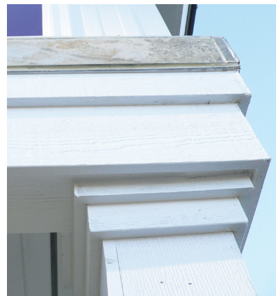
Figure 9. Columns and beams can also be finished with composite trim, which is attached to 2-by blocking fastened to the steel framing (left). Note the tile edge trim detail used to finish the slab (above).
