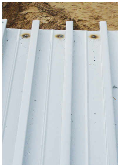
Figure 4. The panels are either screwed or (as shown above) puddle-welded to the steel frame.
