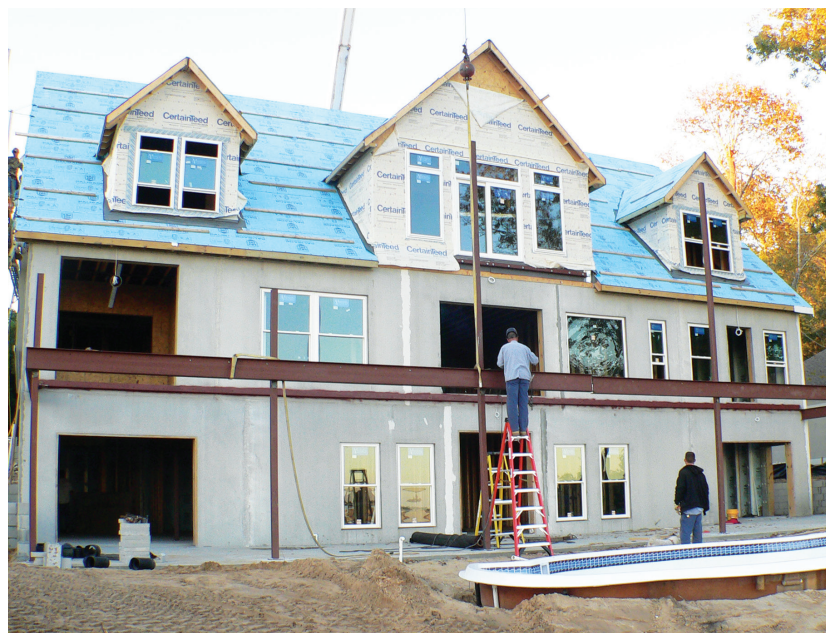
Figure 1. The pans are supported by steel framing (left). The side I-beams are welded to a 5x5 angle ledger that has been through-bolted to the house (above).
