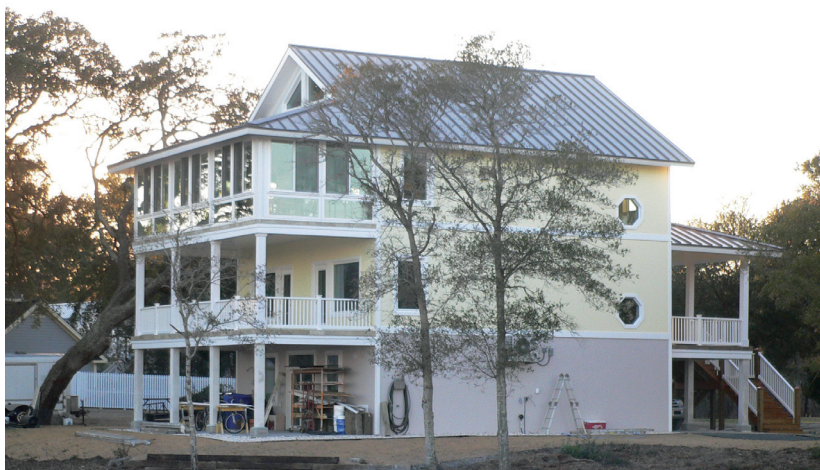
Figure 10. When finished with traditional trim, this coastal home's porches look like they're built with wood, but they are drier and more durable and require less maintenance.
