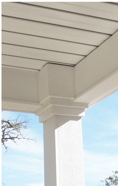
Figure 9. Columns and beams can also be finished with composite trim, which is attached to 2-by blocking fastened to the steel framing (left). Note the tile edge trim detail used to finish the slab (above).
