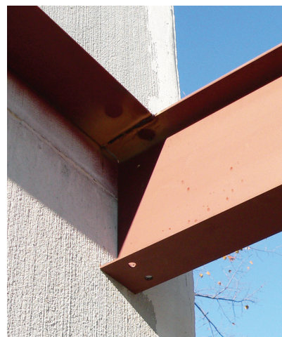
Figure 1. The pans are supported by steel framing (left). The side I-beams are welded to a 5x5 angle ledger that has been through-bolted to the house (above).
