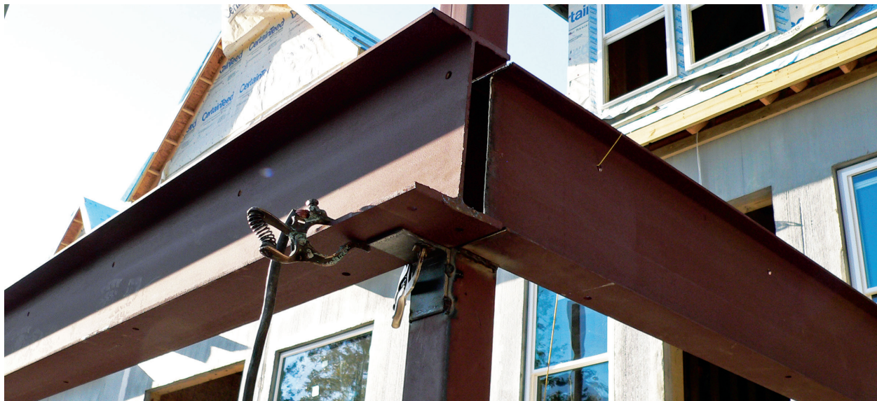
Figure 2. Around the perimeter of the deck, the I-beams that support the panels are welded to 4x4 steel columns.
