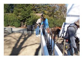
ICFs typically have an intricate network of rebar and webbing that concrete must flow around to fill the forms properly.
