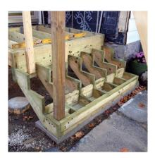
Instead of framing stairs one piece at a time, I like to prefabricate stringer "kits." Not only does this technique speed up the job and improve accuracy, it allows me to assemble the components on a work table rather than while kneeling in the dirt.
