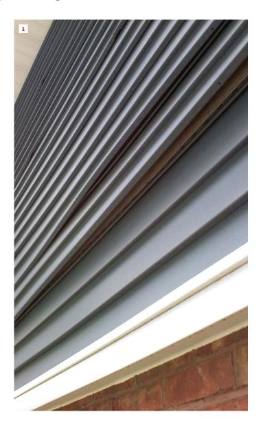
In older two-story homes with vinyl siding, it's common to see siding panels that have uncoupled between floors. Shrinkage in the structure behind the siding is most likely the cause.
