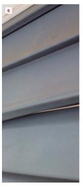
There are two different ways to reconnect separated panels. The first method is cutting a strip off a metal starter strip and inserting it into the lower locking strip (2). The second method is cutting the face off J-channel and inserting that into the locking strip (3). The unlocking tool then engages the top panel with the newly-added strips (4, 5).
