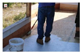
"kick" more quickly. Smaller batches ensure that the resin does not begin curing before it is applied.
