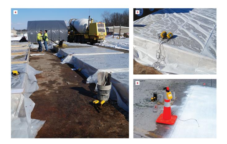
to cold winter air, posing a major risk of damage due to early-age freezing. So research is ongoing to justify the application of maturity methods to exposed flatwork in cold weather conditions.
