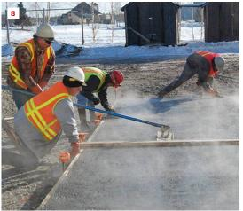
Above: A crew from a local concrete contractor in Fairbanks, Alaska, places concrete slabs in freezing weather at nearby Fort Wainwright, raking out the concrete (7) and bull-floating it (8), just as they would in summer weather. CRREL researchers report they have designed freeze-resistant concrete mixes that can be handled, placed, and finished just like typical mixes, even in very cold weather.
