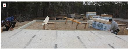
The first line is for the longest wall, or baseline wall, of the house. Using a gauge block made from the plate stock, draw inside corners at both ends of the wall (1). Check the measurement to confirm that the wall length is correct, then snap a line between the corners. From both ends of the baseline wall, measure out for the longest parallel wall (which establishes the largest rectangle on the floor deck), again marking the inside of the gauge block (2).
