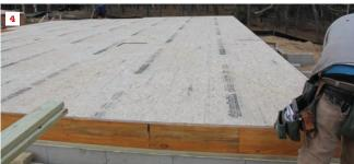
Make an approximate corner mark on one end of the parallel wall and then measure over the length of the wall to mark the corner on the other end. Take diagonal measurements between the corners, first in one direction (3) and then in the other (4).
