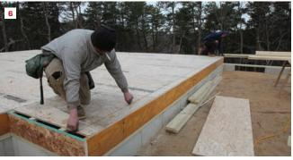
Adjust the corner marks until the diagonal measurements are exactly the same (5). Note that the lighter pencil mark in the photo is the original (approximate) corner mark made before the adjustment. Snap a line between the adjusted marks and the corners of the baseline wall (6). Those walls should be perfectly square to the baseline wall. Lay out the other walls using the established lines as reference and double-checking for square with diagonal measurements.
