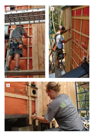
For a reverse board-and-batten cladding, the thin battens are nailed onto the wall first, and the wider boards are nailed over them, so the battens are behind the gaps (1, 2). The method creates an ample space between the siding and the weather resistive barrier, for enhanced drying ability—a significant concern in this deep, superinsulated wall assembly (3).
