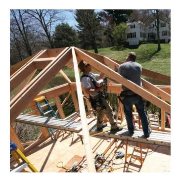
(being careful to keep the four groups together) and cut all the birdsmouths and tails on one side, then on the opposite side. I made my 45° bevel cuts last, getting two jacks from one cut: From the first 2x6, I got the longest jack for one side of the hip and the shortest for the opposite side; from the second 2x6, the second-longest jack and the second-shortest, and so on, stacking the two sides of the hip in two separate piles.
