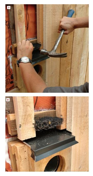
The reverse board-and-batten method creates a substantial air space behind the wood siding, allowing excellent seasonal drying potential. Air inlets behind the horizontal strapping are protected with screening. Gaps between the strapping are protected using Roof Saver vent material, but no screening **(7, 8)**, in order to keep screens from being visible at the spaces between boards.
