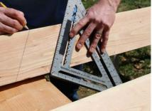
Holding a layout square at a 7:12 angle, the author draws lines representing the long-point plumb cuts where the jacks will meet the hip. He then carries those lines onto the opposite edge of the rafter stock to line up the rafter pattern for the next step of the layout process.
