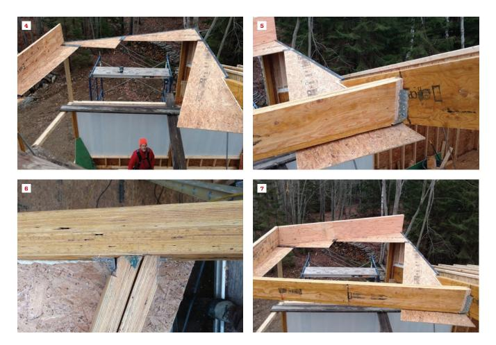
The crew set pie-shaped pieces of Zip System sheathing in place on the skeleton outline of the window-wall structure (4). The valley rafter, downsized to a 12-inch height to allow for insulation above it, had to be shaved at the ends to allow for its out-of-square and out-of-level orientation with respect to the common rafter supporting it at the uphill end, and the wall header supporting it at the downhill end (5, 6, 7).
