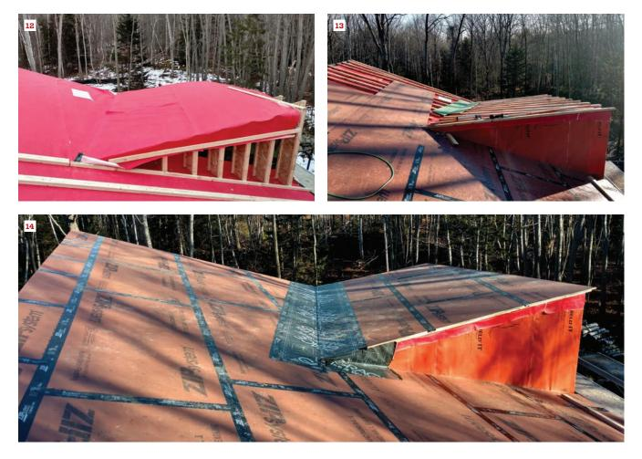
With the roof framing complete, the crew constructed a vented roof assembly. Vapor-open, water-resistive VaproShield SlopeShield roof membrane was attached to the rafters (12), and 2x4 furring laid on top of that. Then the crew sheathed over the furring with Zip System roof sheathing (13), sealing the seams with Zip tape and protecting the valley with Grace Ice & Water Shield (14). The 16-inch I-joist rafter cavities would later be filled with dense-blown cellulose insulation.
