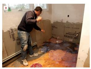
This floor was out of level by a full inch in one direction (1), and by 3/4 inch in the other (2). Before the leveler can be mixed and poured, the author applies liquid primer to the underlayment (3).
