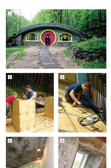
The hobbit home's front facade **(1)**. Georgia and Jude Costigan build one of the home's four skylight-well forms **(2)**. Terence Costigan installs can lighting wired with poly-coated BX cable, both rated to be set in the concrete roof **(3)**. Note the patterns on the finished ceiling in bedroom **(4)** and skylight well **(5)**.
