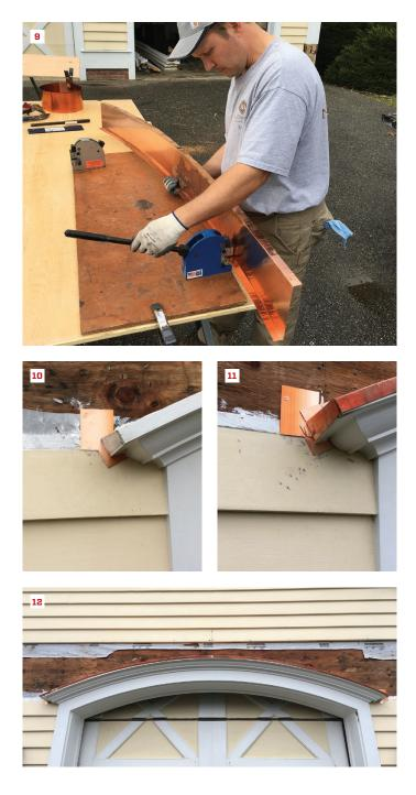
Flashing was shaped with Eastwood shrinker (blue) and stretcher (gray) tools (9). Flashing in the corners helps direct water away from the wall (10). Flashing was installed with minimal nailing; ends were folded down (11). The center seam was soldered (12).
