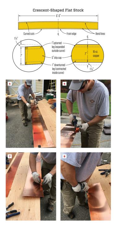
The author laid a crescent-shaped template on wider copper stock (5), traced the slight curve, and cut it out with snips (6). He used a scribe block to mark the 1-inch fold line for the flashing's downward vertical leg (7) and then used a hand brake to bend the leg (8). He repeated the process for the upward leg.
