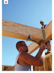
The author positions the first doubled LVL **(5)**. Once these first pieces are nailed off, the telehandler becomes a work platform for laminating the third **(6)** and fourth layers **(7)**. The telehandler supports the beam while end support is installed **(8)** and the structural assembly is secured with a beam hanger **(9)**.
