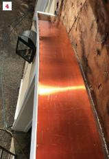
At top are the repaired carriage-house wall and arch-top garage doors (1). Water damage was due to a poorly flashed drip cap (2). The sloped drip cap made a tricky flashing job even trickier (3). The copper overhung the cap in the center when laid in place; the flat stock needed to be crescent-shaped to fit properly (4).
