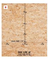
The first course starts with a snapped line to keep the course straight (6). A crew member drops a sheet into place, using one foot to keep it from sliding away (7). A sledgehammer and block drive the sheets together (8). Spacing instructions are printed on every sheet (9).
