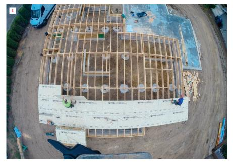
At right is a bird's eye view of the floor sheathing process. A crew of two works in harmony to sheathe this floor quickly and efficiently. The crew member on the right spreads glue on the joists while the crew member on the left takes sheets from the stack, drops them into place, and tacks them on layout. When the glue is spread for one course, the person gluing will take over dropping and tacking while his partner fastens the sheets with a screw gun.
