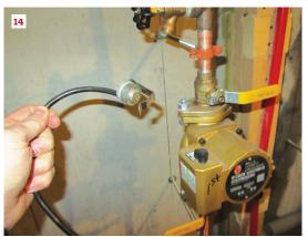
When a large house is served by a well with possibly limited water production, large buffer tanks (12) can ensure that water does not run out during high-demand periods. Recirculating timers can go out of synchronization, in the author's experience (13). One way to reduce wear on recirculation lines is to use an aquastat (14) that turns the pump off when the line is hot.
