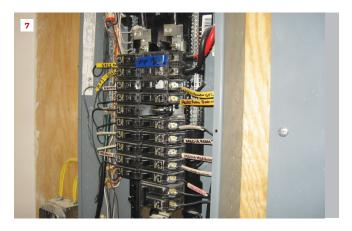
When power circuits and lighting-control circuits are extensive enough to fill several panels (5), it can be helpful to organize some circuits into sub-panels located around the building (6). Every circuit should be clearly labeled to indicate what it's for and where it leads (7).
