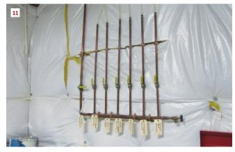
A manifold system (8) is a good way to keep dozens of hot- and cold-water runs organized. The author recommends organizing outdoor-hose-bibb piping lines and gas lines at a central location (9, 10, 11), with the capability of shutting all the lines down at once as well as individually, and with all lines clearly labeled to indicate what they serve and where they terminate.
