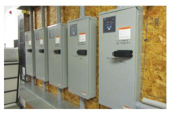
The wiring circuits for a huge house (1, 2) can pose a challenge to installers and to maintenance or remodeling companies. The author recommends terminating wiring runs in panels in a way that will make sense to the owners and future electricians (3, 4), and labeling every wire with its purpose and the location of the devices or receptacles it serves.
